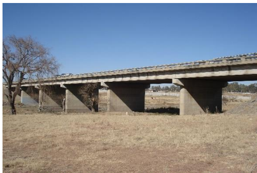
The existing road bridge
