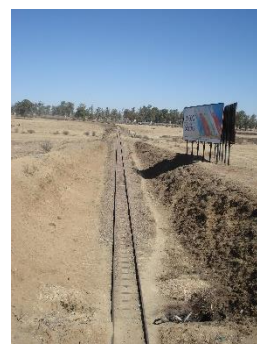
Underpass railroad track
