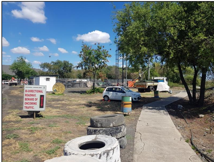
Figure 3-10: View of the project area, looking west towards the storage yard across a small lawn.
