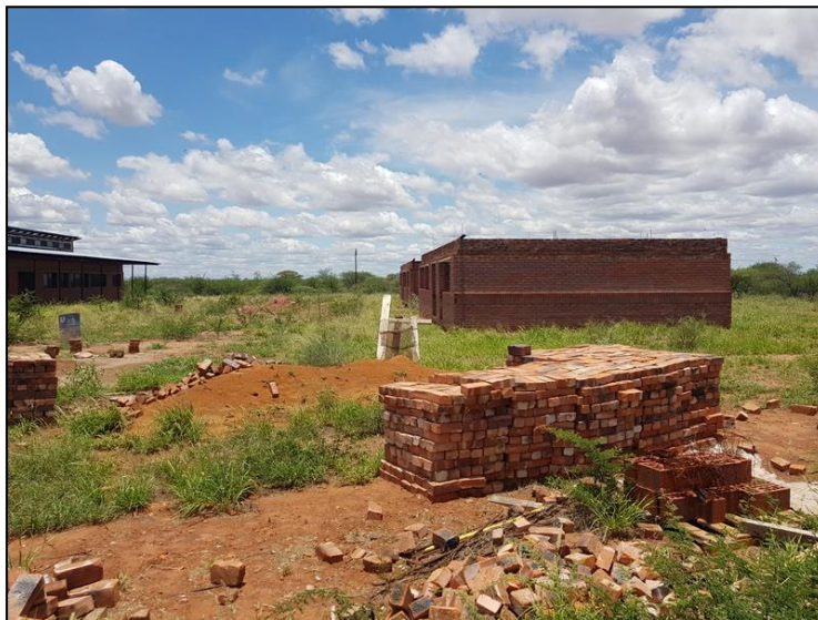
Figure 3-4: View of partially completed additional offices in the project area.
