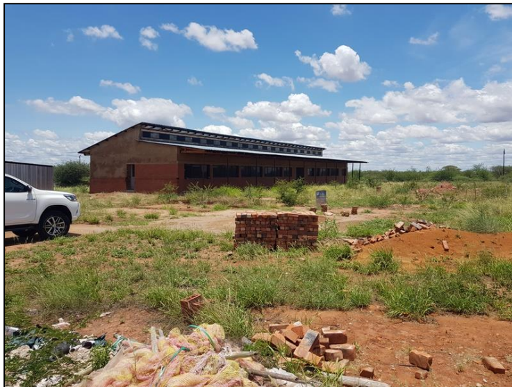
Figure 3-3: View of partially-completed offices in the project area.
