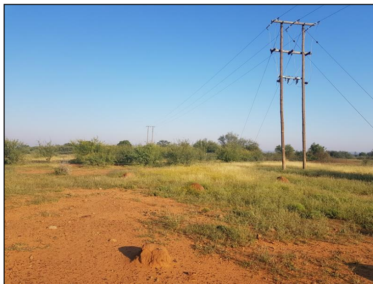
Figure 3-1: View of a powerline bisecting the project area to the north.
