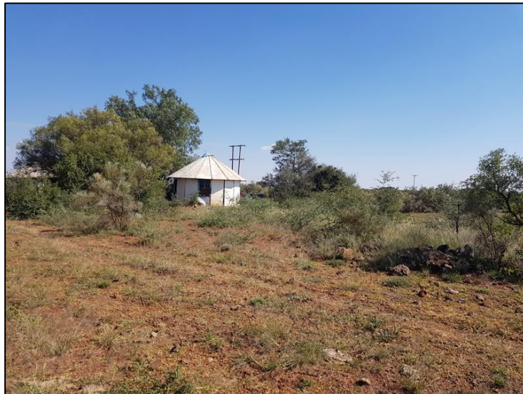
Figure 3-9: View of temporary structures at the farmstead compound south of the project footprint.
