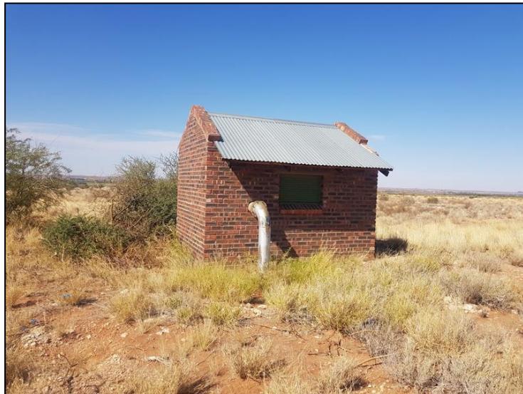
Figure 3-4: A small modern pump house present in the project area.
