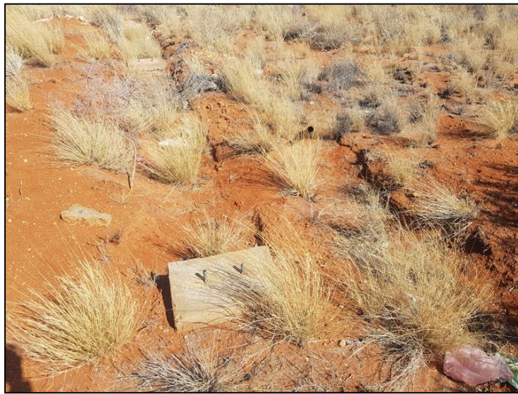
Figure 3-3: View of concrete foundation structures and trenches in the project area.
