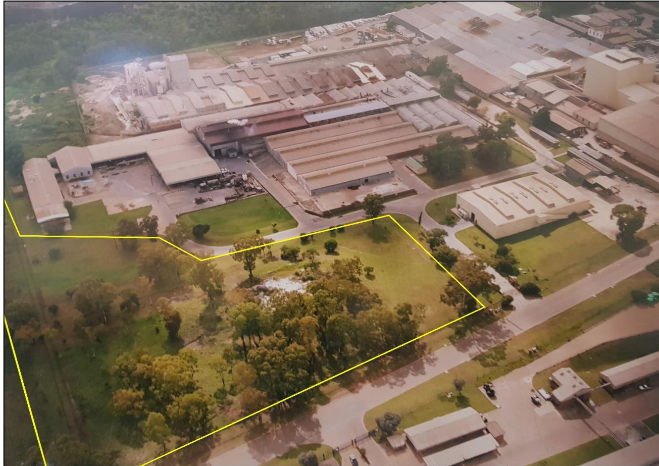
Figure 2-3: High Resolution aerial image of the A-Thermal Retort Technologies Plant. The upgrade project area is partially indicated in yellow line.
