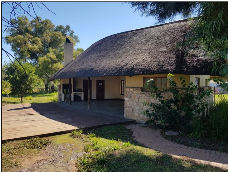
Figure 3-9: A recreational building in the bird sanctuary within the project footprint areas.
