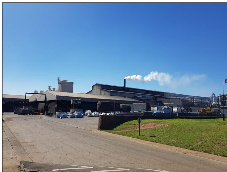
Figure 3-3: View of the A-Thermal Retort Technologies Plant north of the project area.
