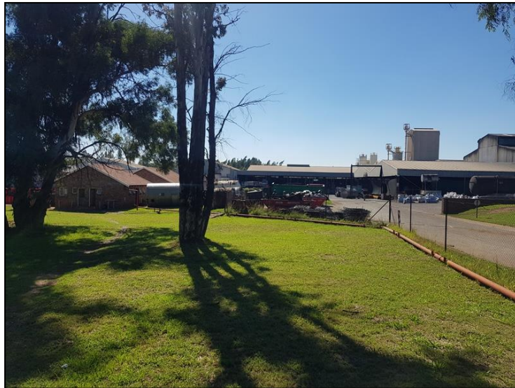
Figure 3-2: View of a lawn in the project area, the existing A-Thermal plant is visible in the distance.
