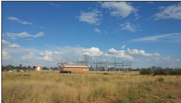
Figure 3-8: View of the Umtu Substation and the southern offset of the proposed corridor.
