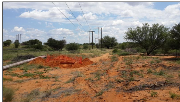
Figure 3-5: View of sands and degraded surface cover along a side line connecting to the Hotazel - Heuningvlei ESKOM power line.
