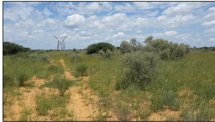
Figure 3-4: View of the study area along the existing Hotazel - Heuningvlei ESKOM power line near the town of Hotazel.
