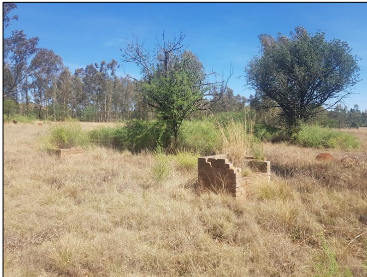
Figure 3-9: Partially destroyed braai structures in the project area.
