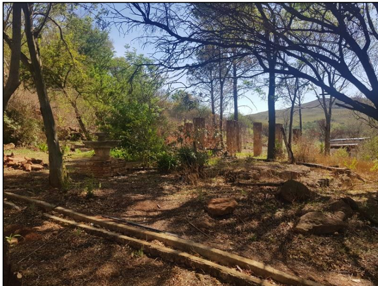
Figure 3-15: The partially collapsed remains of a water fountain (left) and a concrete hedge at the modern residence.
