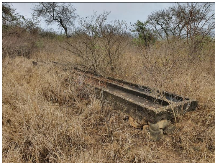
Figure 5-15: View of a livestock drinking trough at Site Exigo-BOD-HP03.
