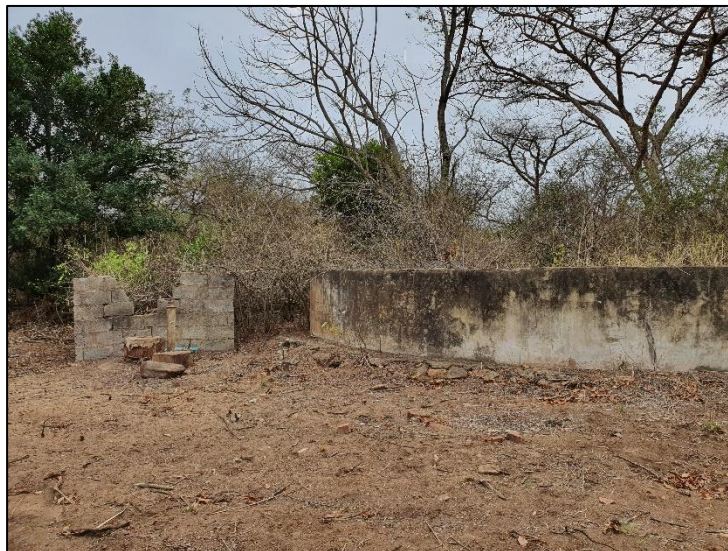
Figure 5-8: View of the disused concrete dam at Site Exigo-BOD-HP01.
