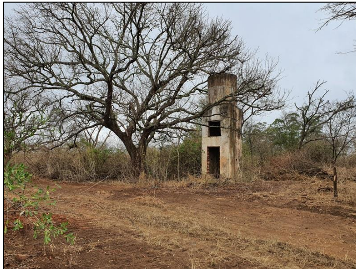
Figure 5-14: A water tower at Site Exigo-BOD-HP03.
