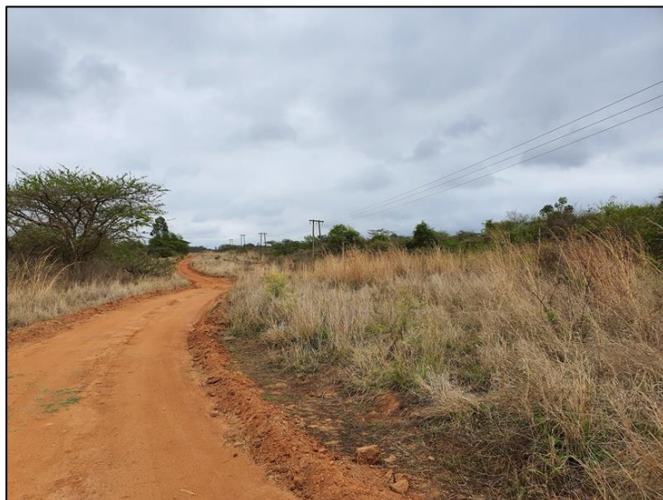
Figure 3-13: The Eskom powerline and servitude bisecting the project area.
