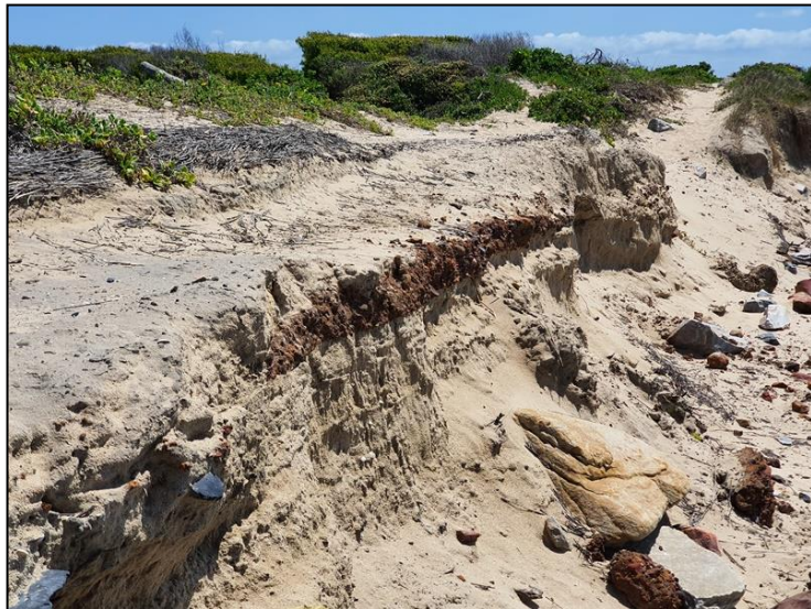
Figure 3-4: Erosion is evident along much of the remaining coastal dunes in the area.
