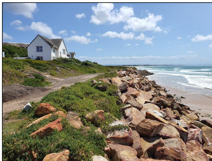
Figure 3-2: View of residential houses and vegetated coastal dunes along rock revetments.
