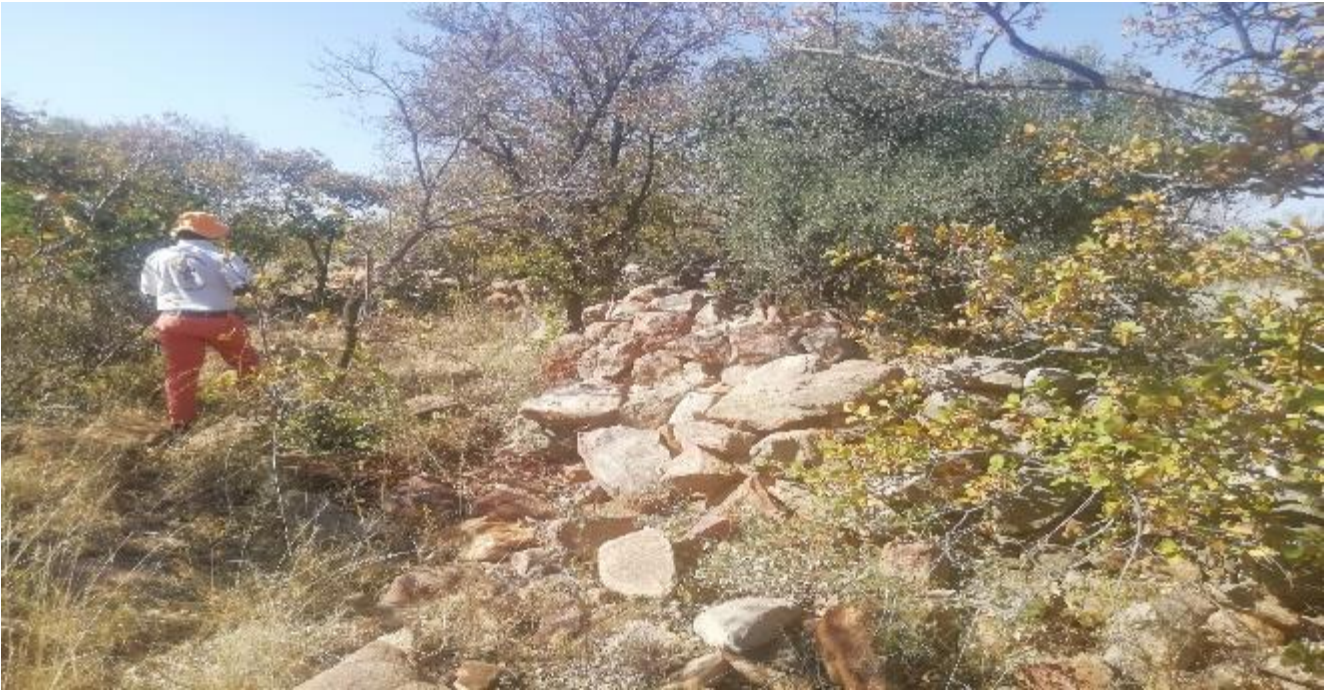
Plate 17: showing a member of the community showing us the collapsed walls.
