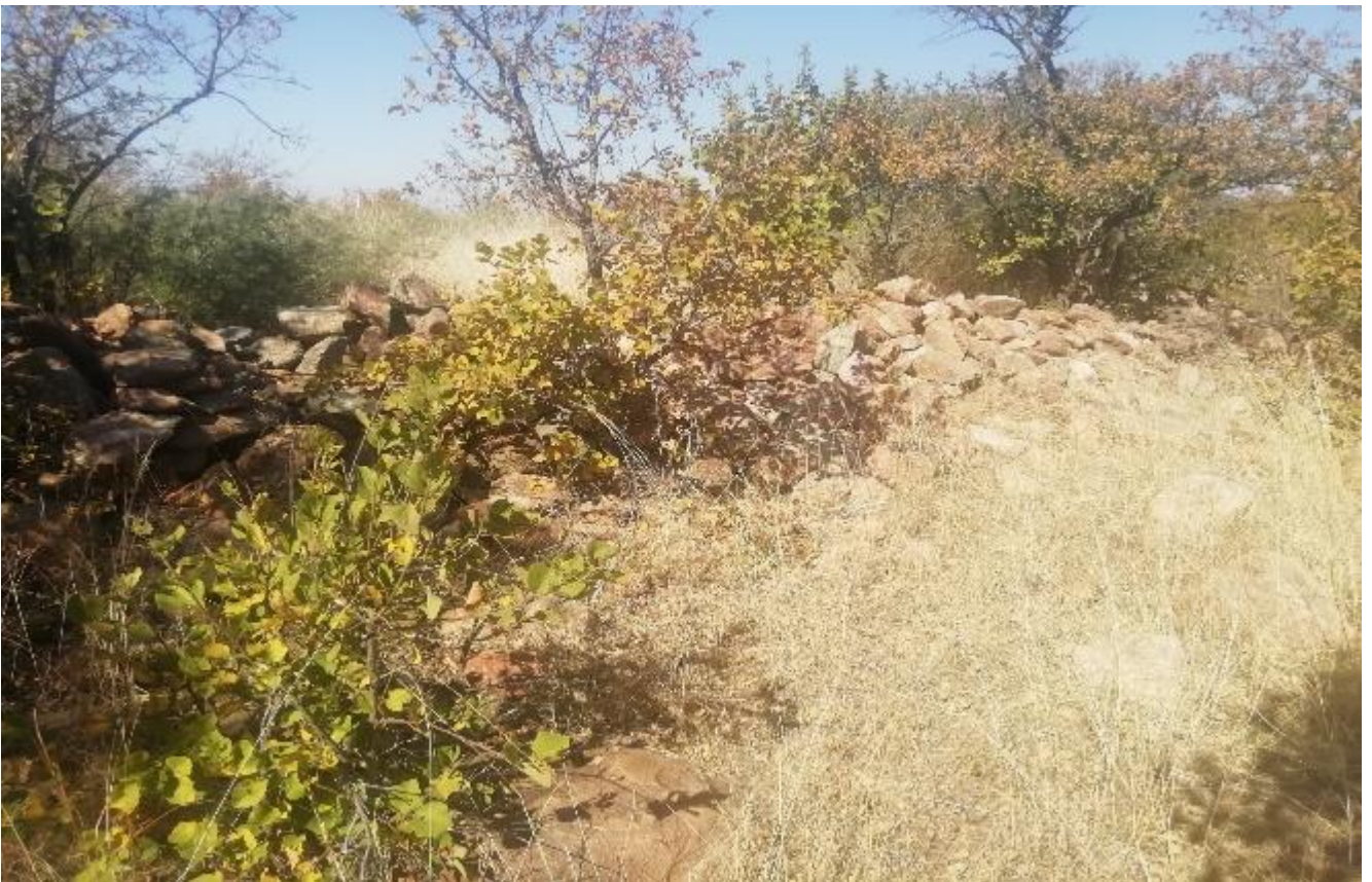
Plate 16: showing collapsed walls at site KSWs-SE2.
