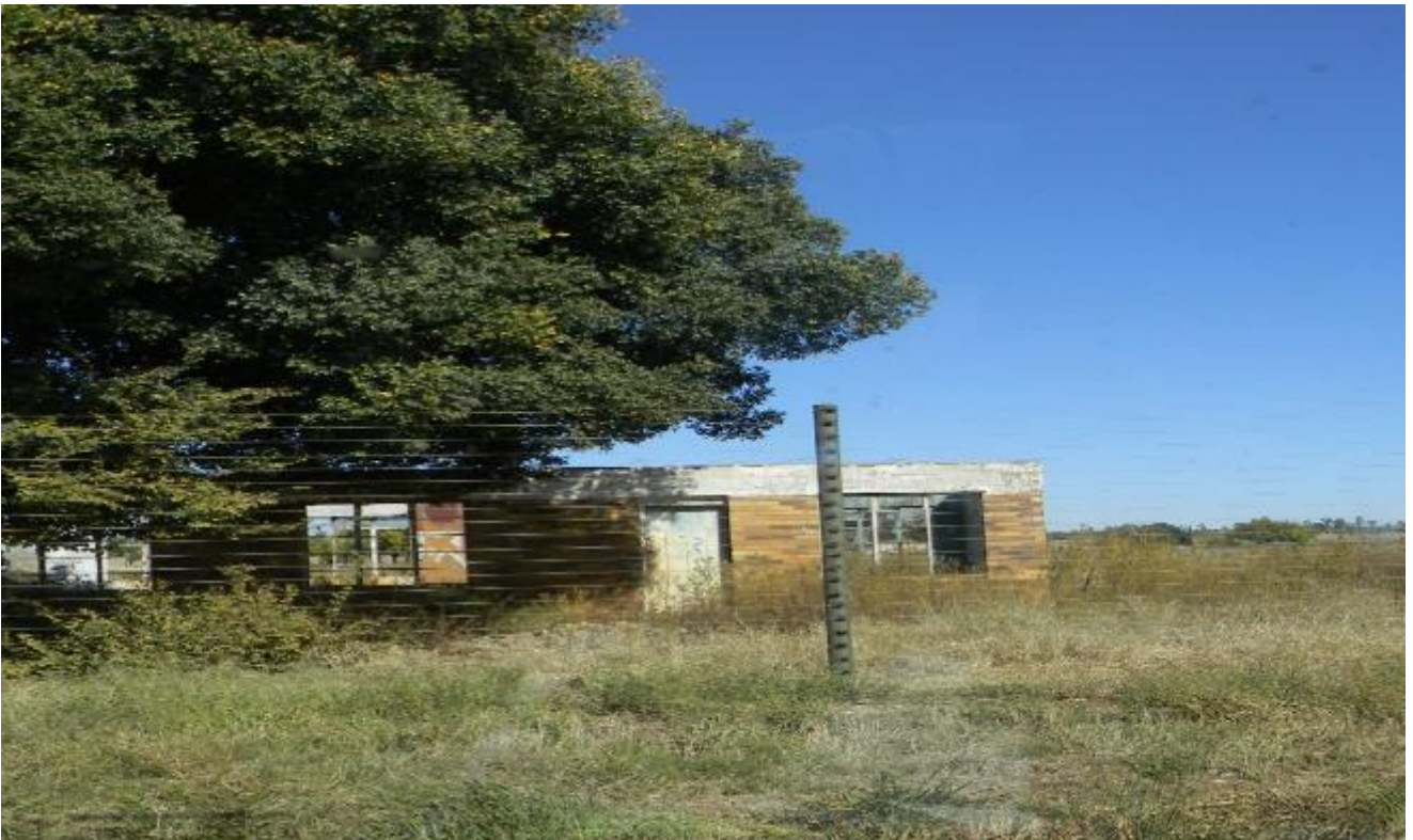
Plate 45: showing abandoned farm buildings within the proposed mining development site.
