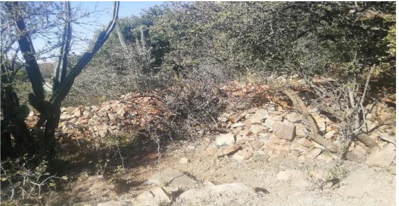
Plate 25: showing collapsed walls at site KSWs-SE3.
