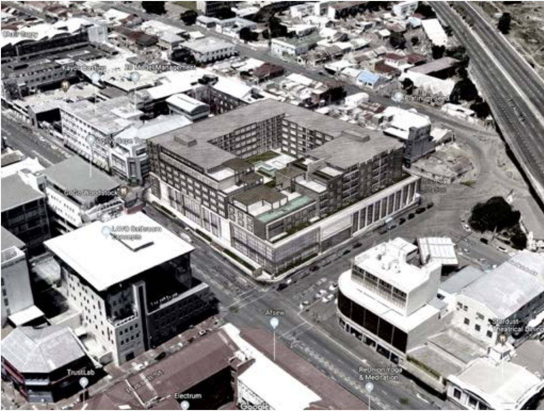
Figure 55: Aerial view of development from north-westerly direction
