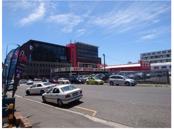
5.14:View of site from Russell Street facing northeast
