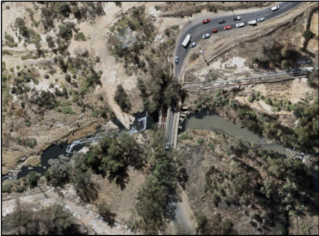
The Old Crownwood Road Bridge, seen from the air (2018) (Image: Google Earth)
