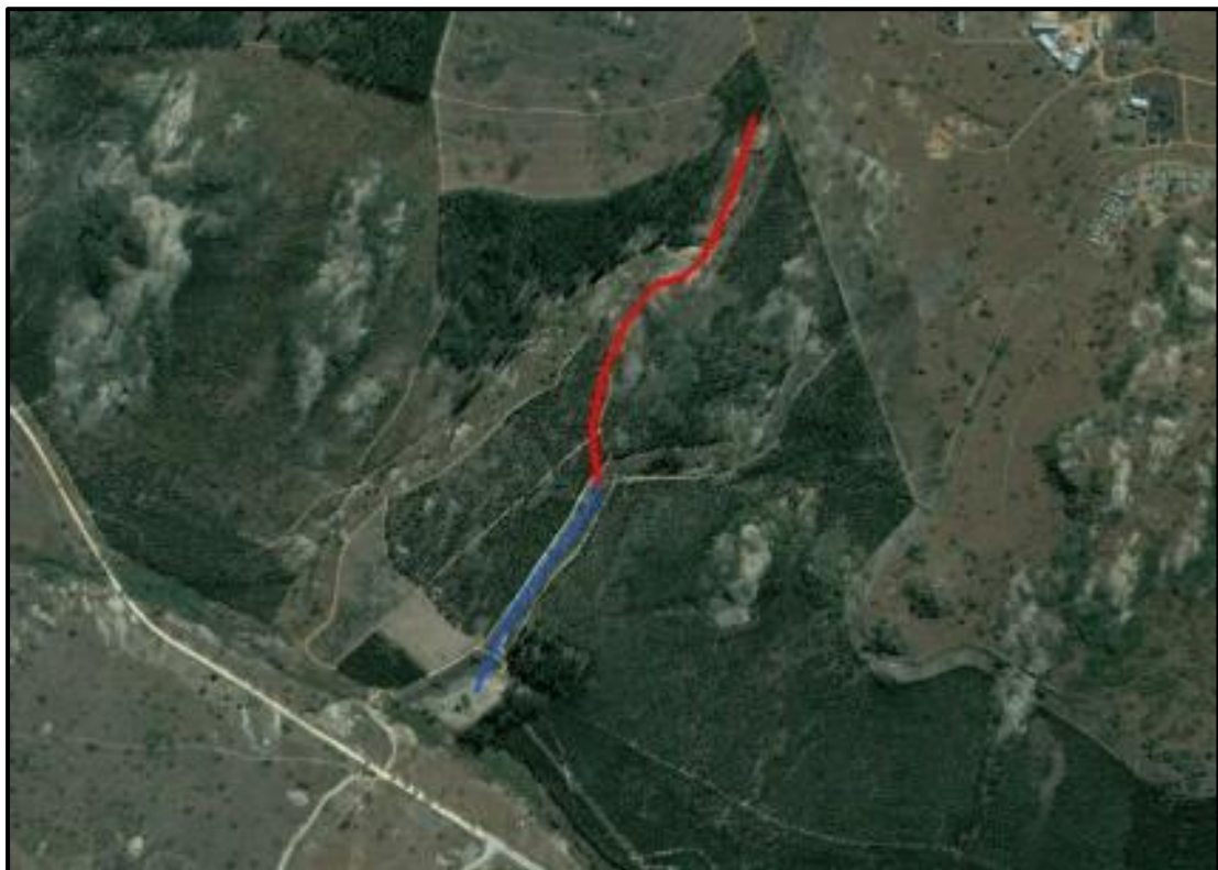
Figure 13. Aerial view of the project area in 2004 (Blue = existing pipeline; red = new pipeline) (Image: Google Earth)
