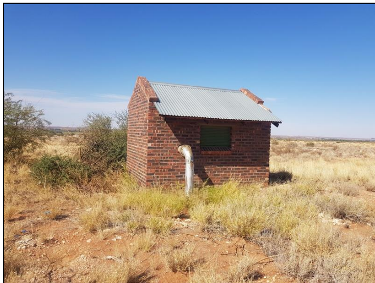
Figure 3-6: A small modern pump house present in the project area.
