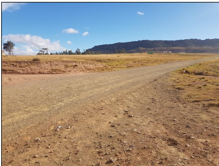
Figure 3-17: View of the western offset of the road upgrade alignment at Lookout.
