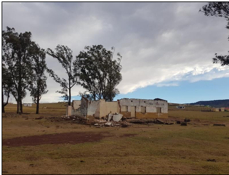
Figure 5-21: View of the remains of the Phillipsdale Trading Store at Site EXIGO-MCRU-HP04.
