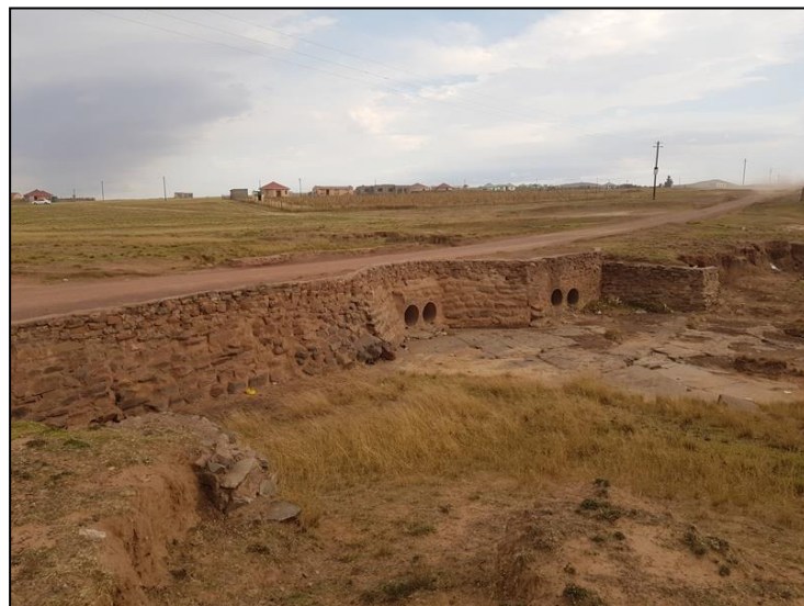
Figure 3-5: View of an existing road culvert in the Singeni area.
