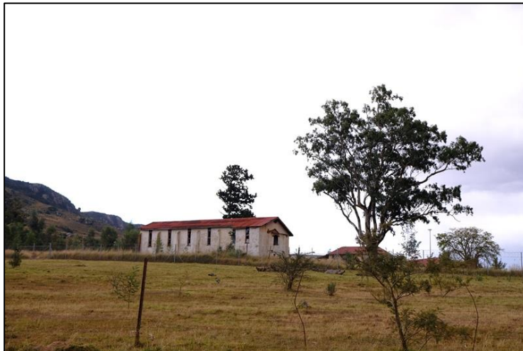
Figure 5-27: View of a building at the Mjanyana Hospital complex.
