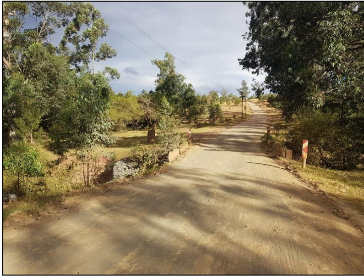
Figure 3-15: View of general surroundings in the project area at Mjanyana.
