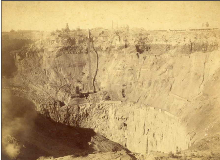
Figure 4-4: Historical photo dating to the last decade of the 19th century, of the big hole excavation at the Kimberly Mine.
