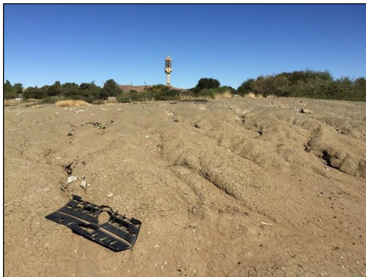
Figure 3-10: View of degraded mine dumping areas along an eastern section of the St Augustine Site.
