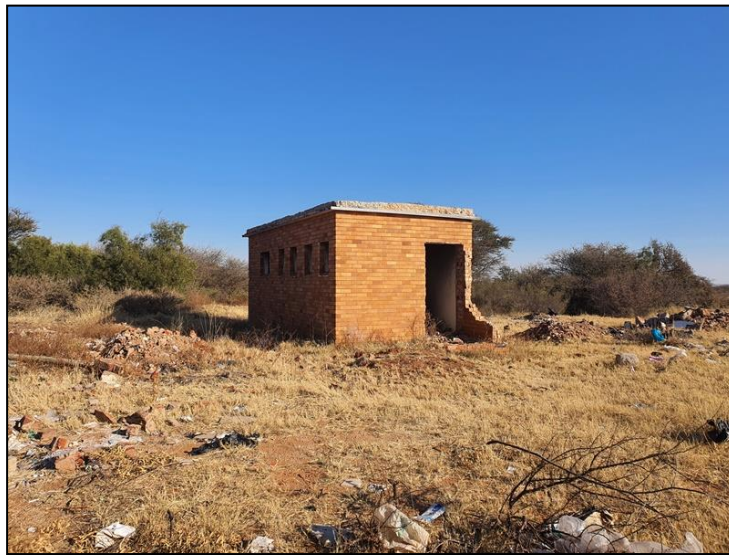
Figure 3-5: View of a small brick building associated with the shooting range.
