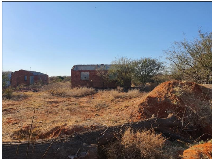
Figure 3-9: View of the remains of a various small dwellings in the project area.
