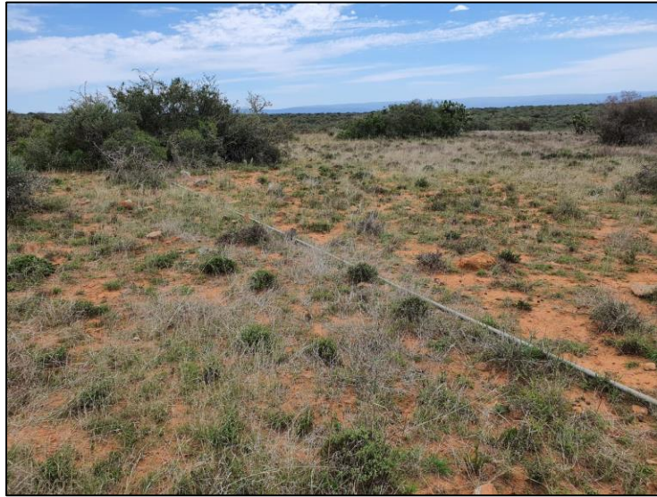
Figure 3-8: View of a water pipeline traversing the project site.
