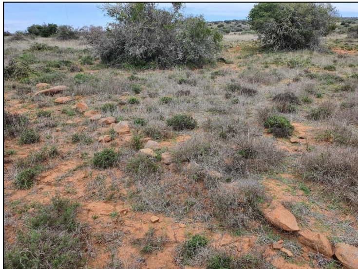
Figure 3-3: View of a water pipeline in the project area, buried with rocks and soil.
