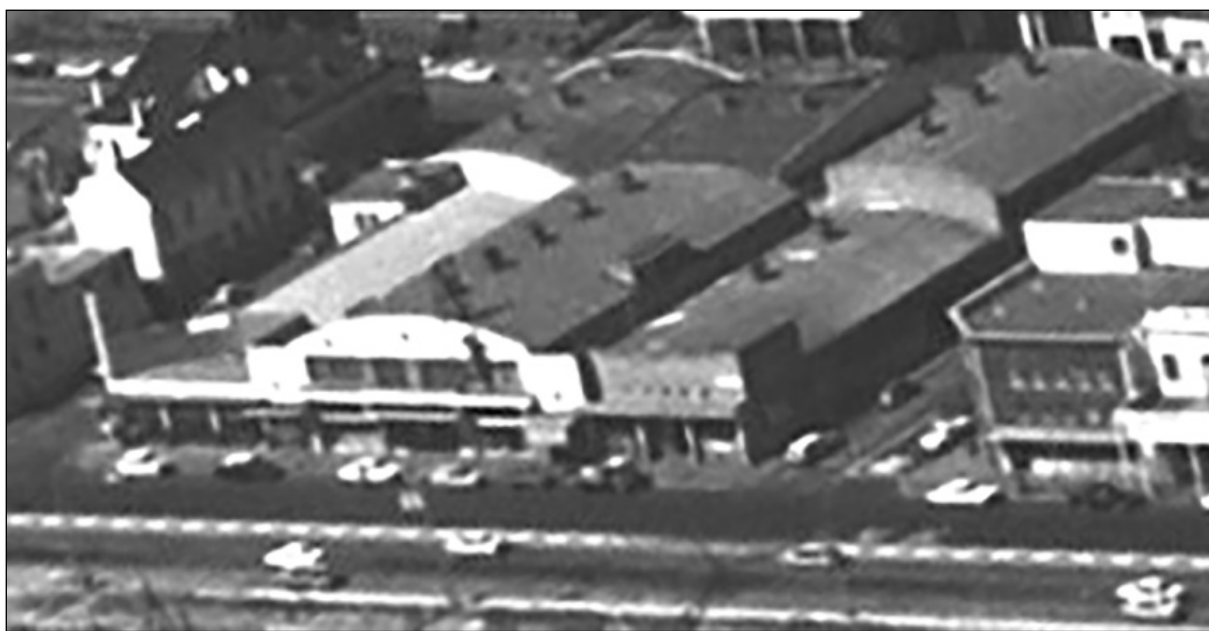
Figure 28: A portion of Figure 6, showing the subject block with Sir Lowry Road seen running along the foreground. By comparing this photograph to Figure 18, it appears that the northern façade has remained relatively intact since the c.1960s, although the upper central windows were painted over at a later date. (CoCT Heritage Office)
