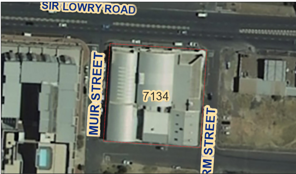
Figure 52: The subject block in 2014, by which time the Oriental Plaza on the west side of Muir Street had been demolished, and the Six-76 Sir Lowry Road building had been erected on the site. Most of the opposite block on the east side of Reform Street had been cleared, but the subject block remained intact. (Chief Directorate: National Geo-spatial Information: 3318CD_19_14_2014_699; annotations by CoCT Heritage Office)
