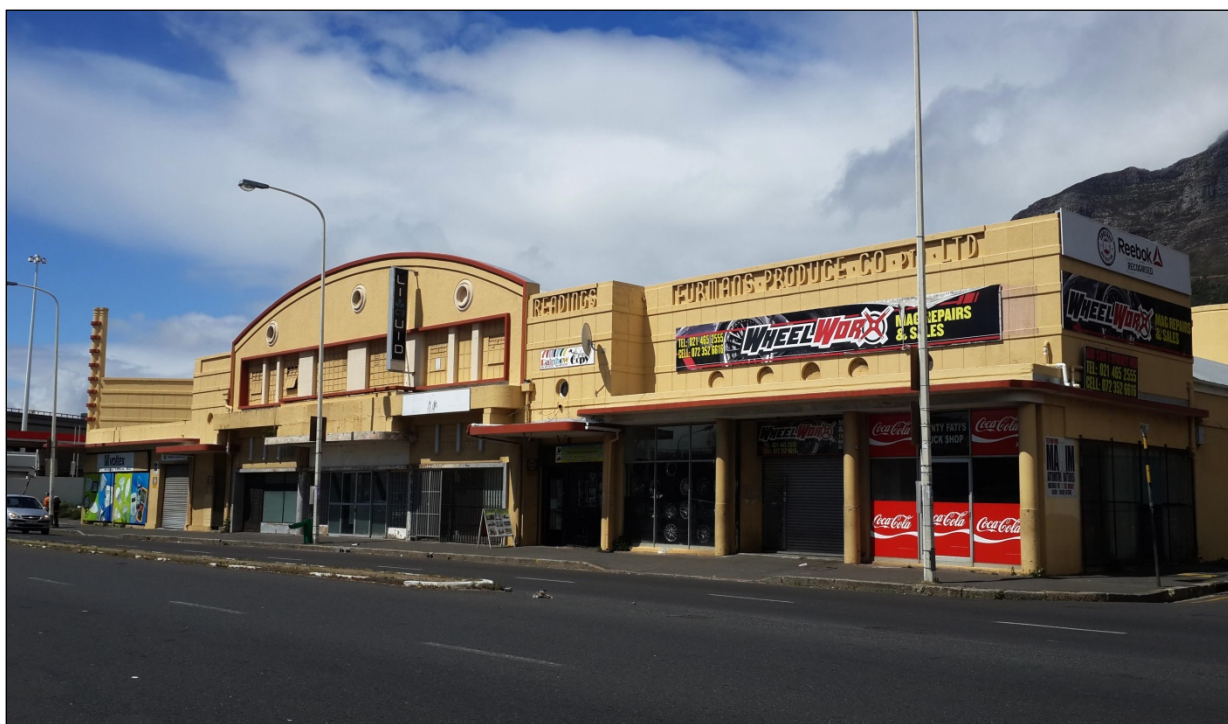
Figure 30: The Sir Lowry Road side of the subject block in September 2014, with the Muir Street edge seen at far right. What is presumably original or early "embossed" signage can be seen on the parapet at right. Furman's Produce & Co. was listed as the tenant in the 1956-7 street directory. The building style was described by Heiko Shulze ( City Bowl Ratepayers' Association ) as "Streamline Moderne, going into International Style". (Jim Hislop)
