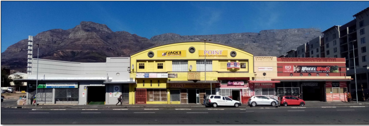
Figure 35: Northern (Sir Lowry Road) façade of the subject block showing new warehouse windows at top centre. (Jim Hislop, 23 April 2021)
