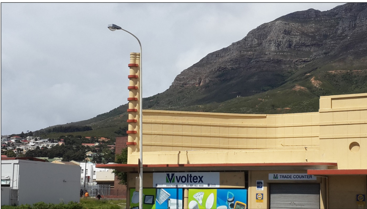
Figure 32: Detail of the eastern parapet in the old filling station/garage section in 2014, which has been closed in since it was built. It would presumably have originally accommodated vehicles undercover. The raised decorative fin is unusual, although two relatively similar fins survive at 21 St John's Street, Gardens. This part of the building has since been occupied by the AVTS Roadworthy Station. (Jim Hislop)
