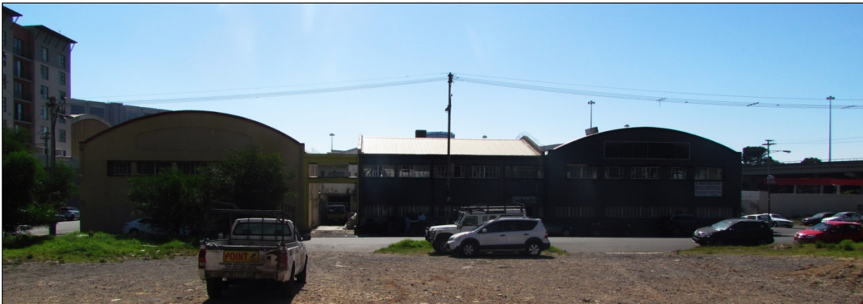
Figure 37: Southern (Selkirk Street) façade of the subject block, seen from the demolished block behind it (Erf 113880), showing the Point Building Supplies vehicle entrance at centre left. (Jim Hislop, 23 April 2021)
