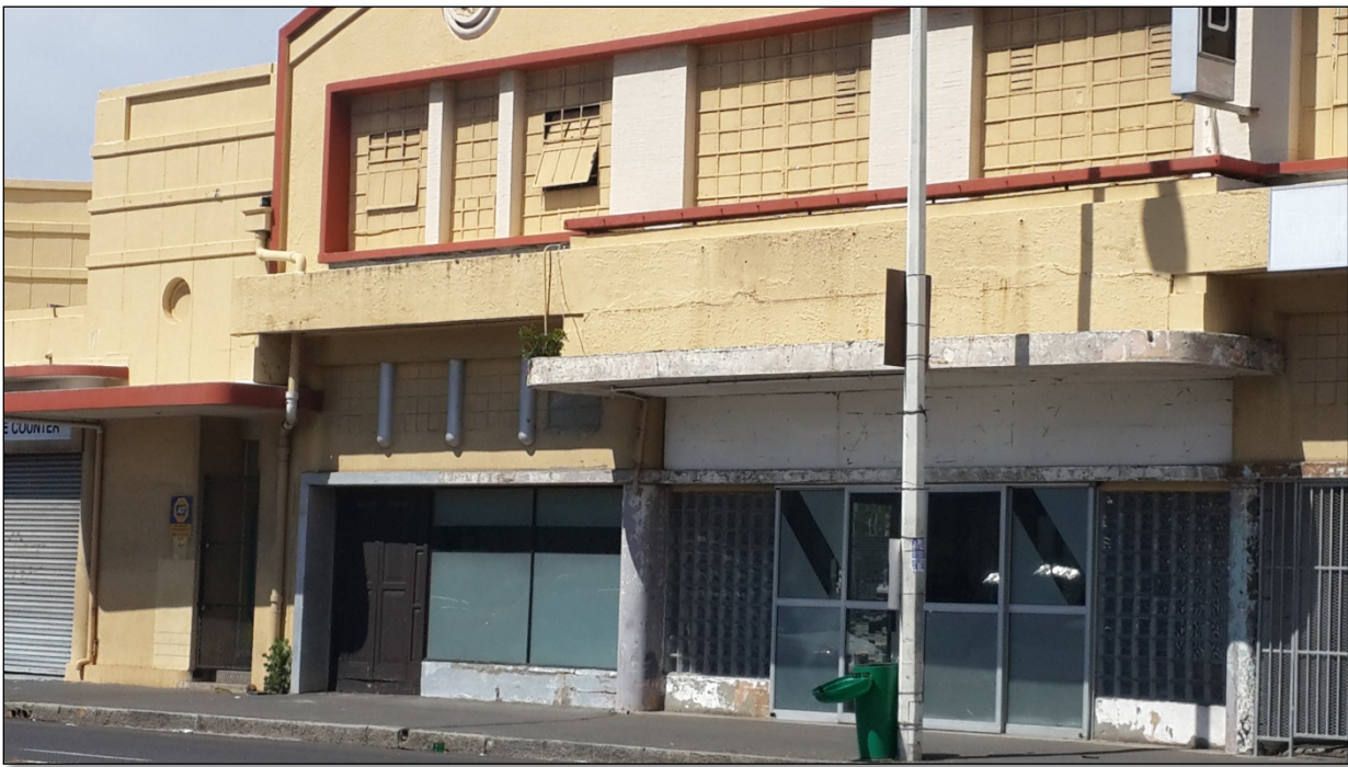
Figure 33: Detail of the altered central entrance portico on the right, already seen with replacement modern doors flanked by glass brick windows, 2014. (Jim Hislop)
