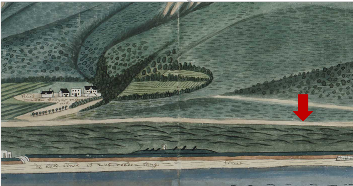
Figure 19: Portion of the Robert Jacob Gordon panorama of c.1778 showing the Zonnebloem homestead and outbuildings to its left on the slope of Devil’s Peak, with open farmland on the right (west). The shoreline can be seen in the foreground, and “The Great Road” (now Sir Lowry Road) can be seen running horizontally below the farm buildings, before its south side was developed with buildings (marked with an arrow). The upper road, seen here above Sir Lowry Road, was presumably the wagon track to Zonnebloem that later became formalised into Hanover Street. (Rijksmuseum, Amsterdam)
