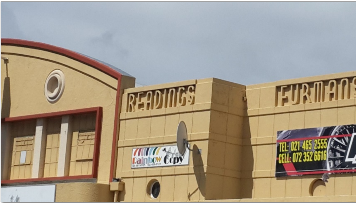
Figure 31: Detail of the western parapet and surviving Furman's Produce & Co. "embossed" signage in 2014. The warehouse windows had been painted over by that time. (Jim Hislop)
