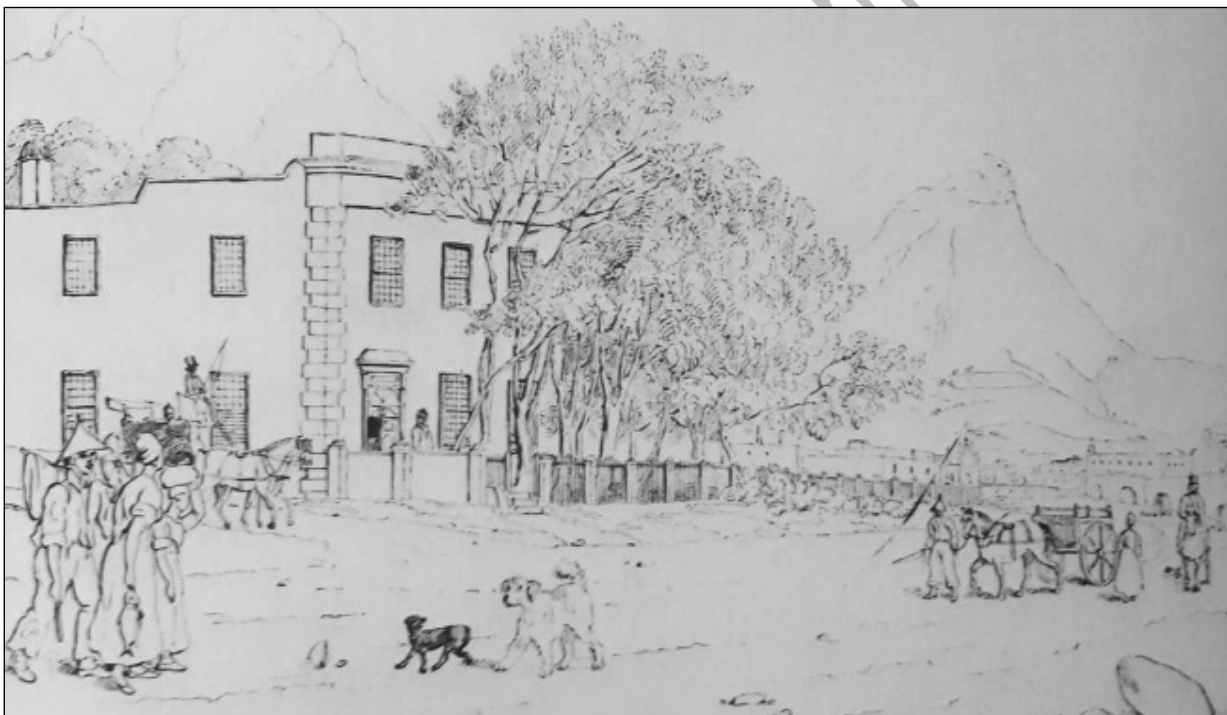
Figure 21: The south side of Sir Lowry Road, looking west towards the Castle in the early 1830s. Gore Lodge, typical of the early 19 th -century double-story merchants' villas that lined the south side of the thoroughfare (not far west from the subject site, and also opposite the Newmarket), was occupied by Sir Charles D'Oyly at the time (the artist of the above drawing). (Western Cape Archives & Records Service: DOY13)
