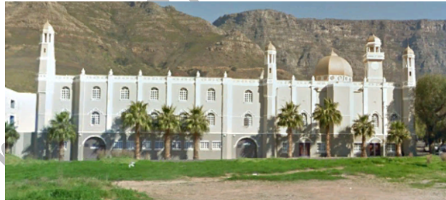
Figure 63: City property, Selkirk Street (GoogleEarth Streetview) Figure 64: Zeenatul Islam Mosque, Chapel Street (GoogleEarth Streetview)
