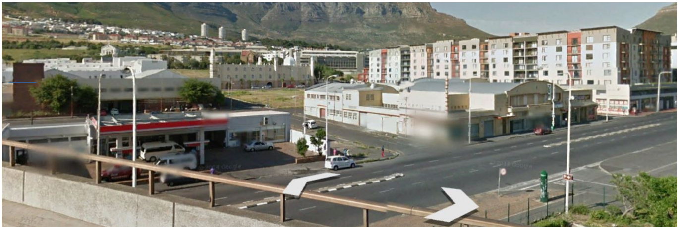
Figure 75: View towards the site from the fly over (GoogleEarth image accessed August 2021)
