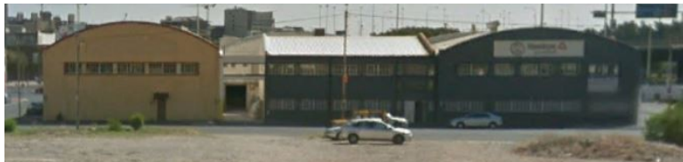
Figure 73: Current Selkirk Street elevation (courtesy Google Streetview accessed October 2021)
