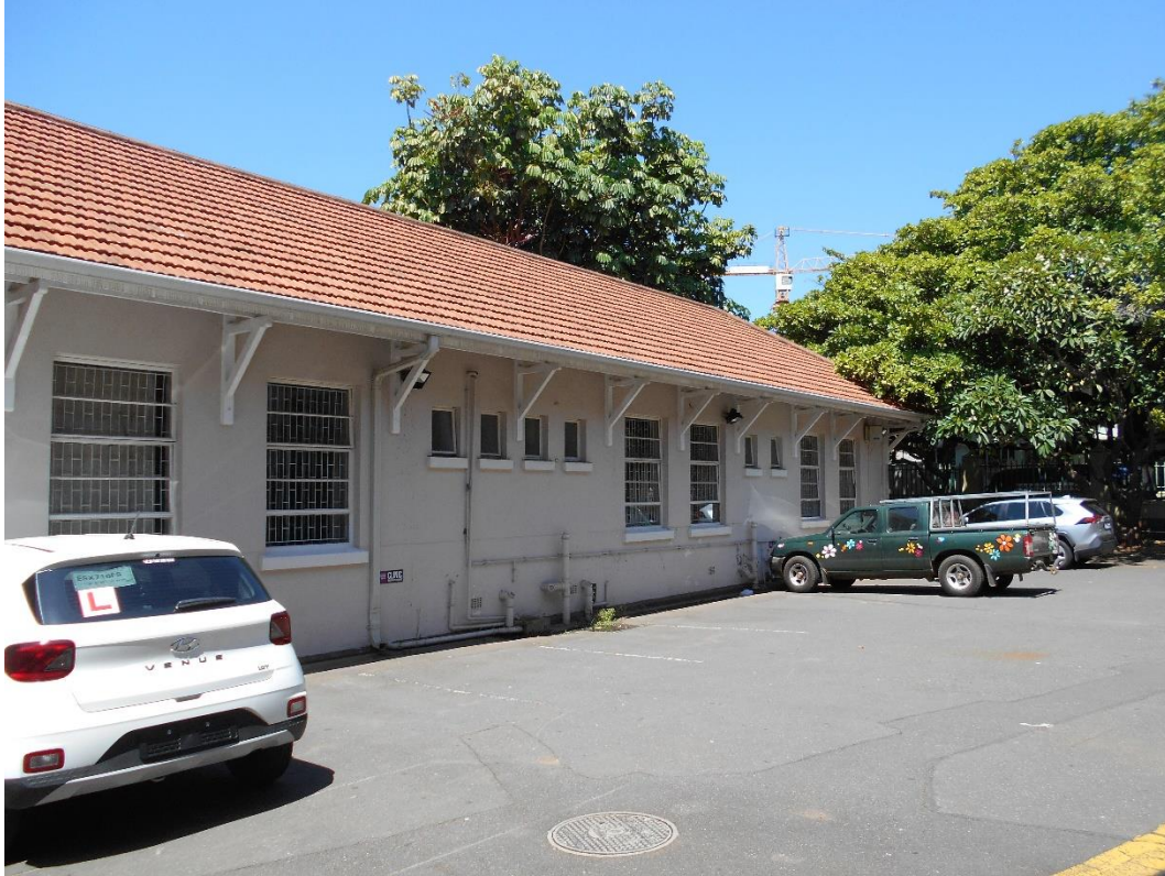
LISTED BUILDING – DUT DRAMA BUILDING
