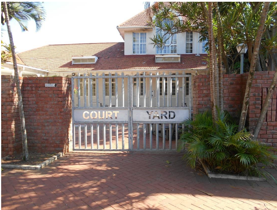
FIGURE 18: ENTRANCE TO THE LISTED BUILDING (AUTHOR)
