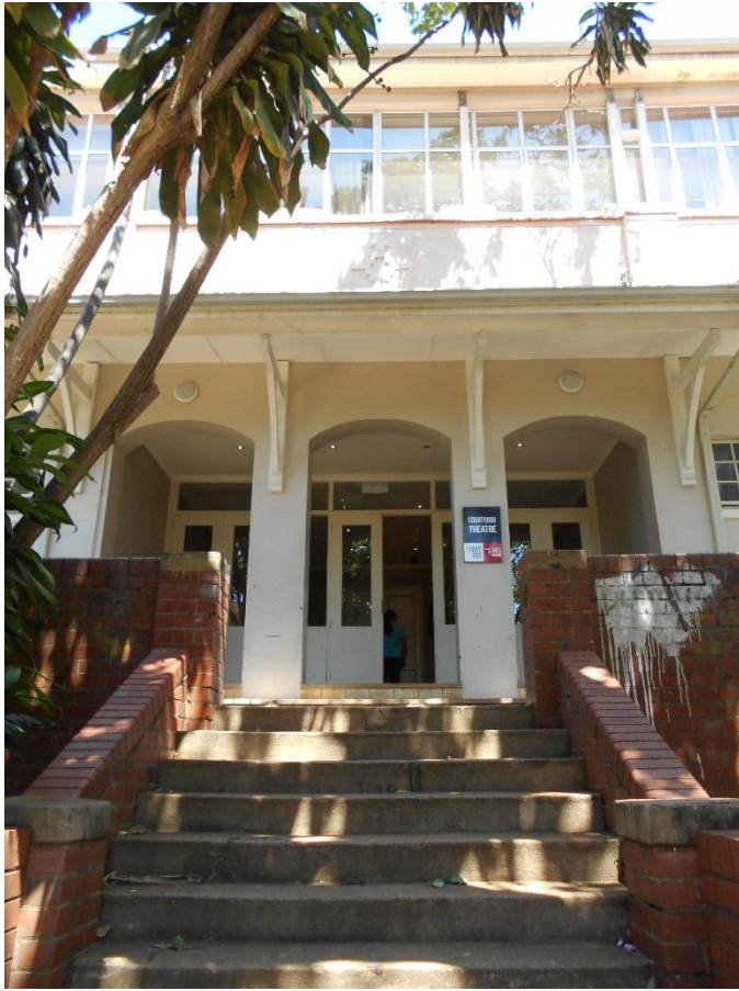
LISTED BUILDING – DUT DRAMA BUILDING
