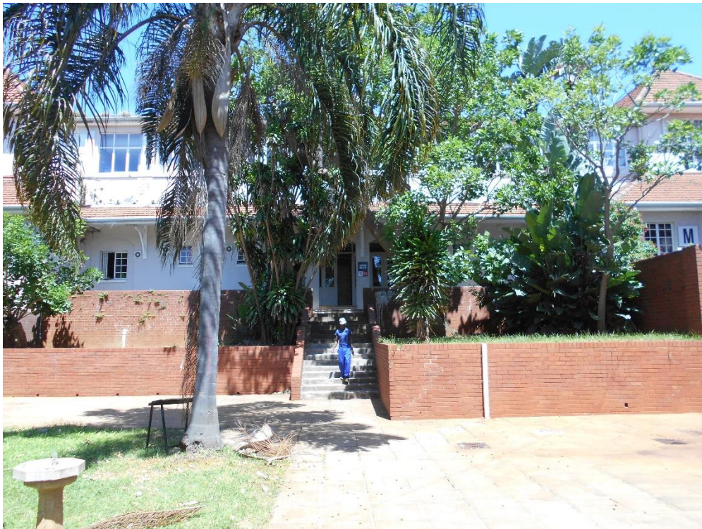
LISTED BUILDING – DUT DRAMA BUILDING
