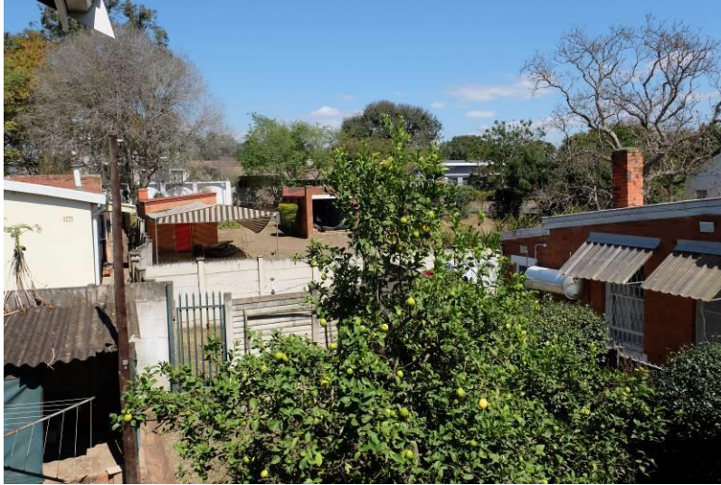
Fig. 29_View from neighbouring property towards the garden side with a number of outbuilding structures (Source: tsica heritage consultants, 22.09.2020)
