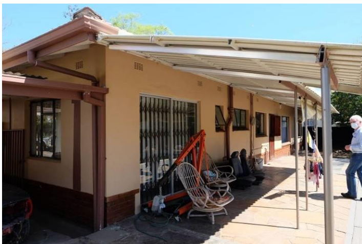
Fig. 58_North-eastern elevation towards the backyard with covered stoep area (Source: tsica heritage consultants, 22.09.2020)
