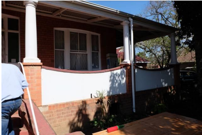
Fig. 17_Verandah roof supported by columns (Source: tsica heritage consultants, 22.09.2020)
