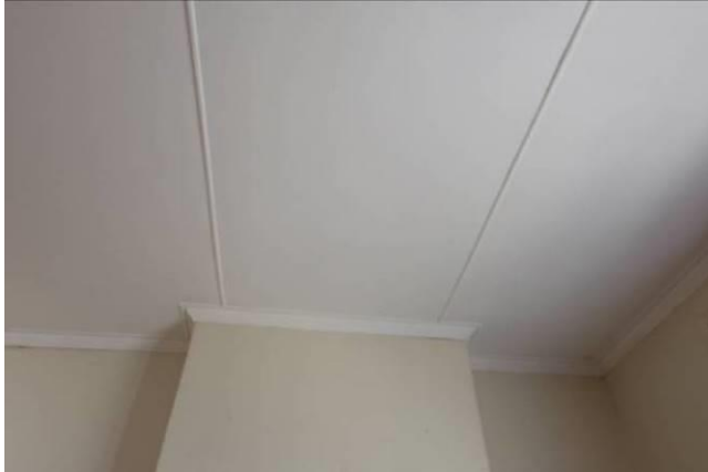
Fig. 67_Original ceiling boards in lounge area (Source: tsica heritage consultants, 22.09.2020)
