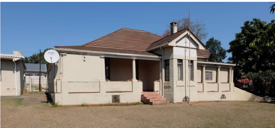
Fig. 116_Typical historical residence from around 1910 with front verandah supported by columns with newly added roof tiles (Source: tsica heritage consultants, 22.09.2020)
