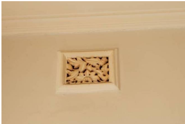
Fig. 68_Original air vent with floral pattern (Source: tsica heritage consultants, 22.09.2020)
