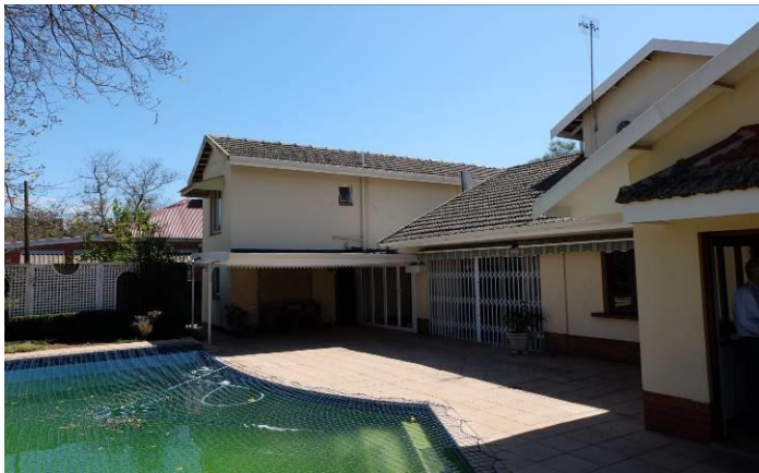
Fig. 43_South-western elevation towards the swimming pool (Source: tsica heritage consultants, 22.09.2020)
