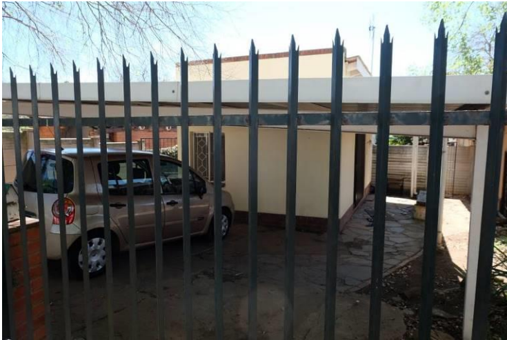
Fig. 60_Single storey building structure on Ptn 68 of Erf 498 used as cottage (Source: tsica heritage consultants, 22.09.2020)
