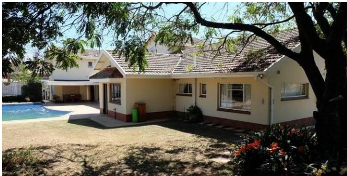
Fig. 41_South-western elevations towards garden and swimming pool (Source: tsica heritage consultants, 22.09.2020)
