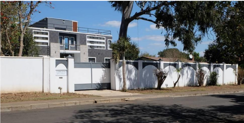
Fig. 111_View along Carbis Road in western direction with newly built double storey residence (Source: tsica heritage consultants, 22.09.2020)
