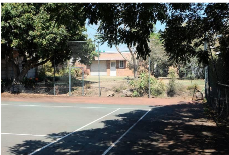
Fig. 49_View towards in south-western direction with single storey outbuilding located along Carbis Road (Source: tsica heritage consultants, 22.09.2020)
