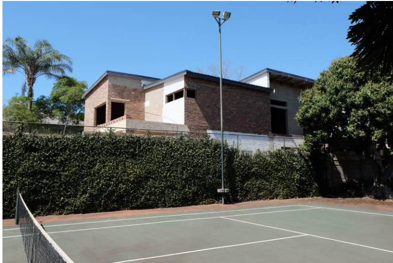
Fig. 47_View towards the neighbouring property in south-eastern direction, fence of the tennis court forms boundary of the property (Source: tsica heritage consultants, 22.09.2020)
