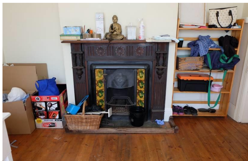
Fig. 64_Original fireplace and wooden floor boards in bedroom (Source: tsica heritage consultants, 22.09.2020)
