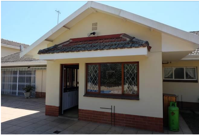
Fig. 44_Entrance to the kitchen along south-western elevation towards the swimming pool (Source: tsica heritage consultants, 22.09.2020)
