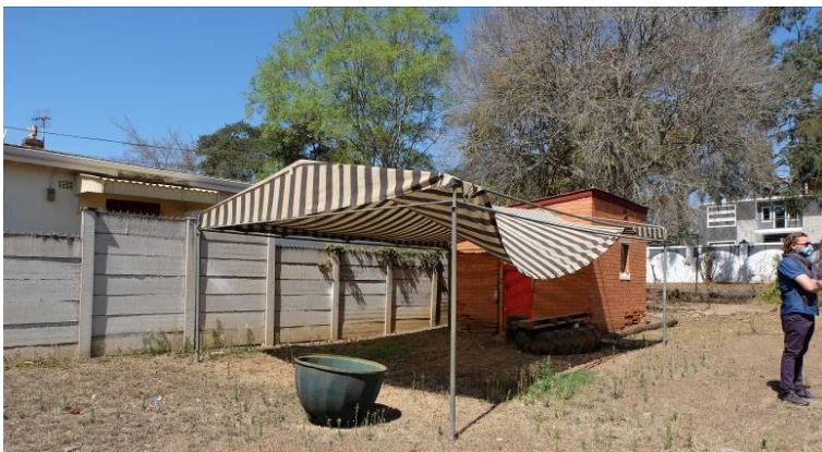
Fig. 63_View towards north-western boundary line from Ptn 68 of Erf 498 with single storey building structure located along the boundary wall (Source: tsica heritage consultants, 22.09.2020)
