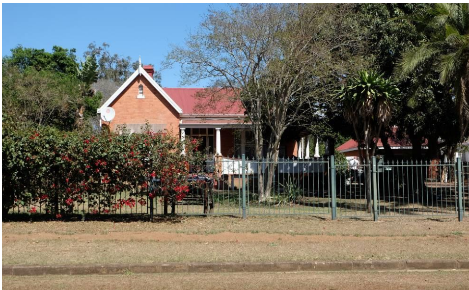
Fig. 9_Street elevation with main entrance to Roseveare Road, single storey red brick and corrugated roof residence with triangular gable and corner verandah supported by columns (Source: tsica heritage consultants, 22.09.2020)
