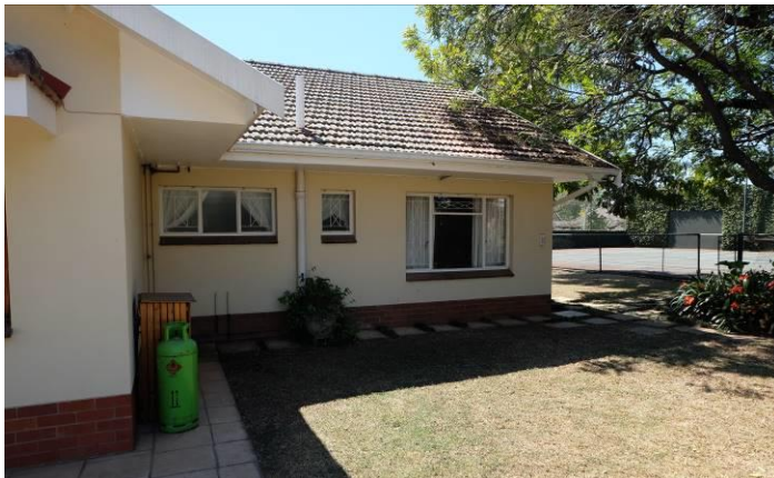
Fig. 42_South-western elevation towards garden and view towards the tennis court side (Source: tsica heritage consultants, 22.09.2020)
