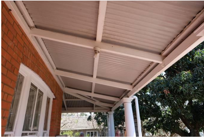
Fig. 21_ Verandah roofing with wooden trusses (Source: tsica heritage consultants, 22.09.2020)
