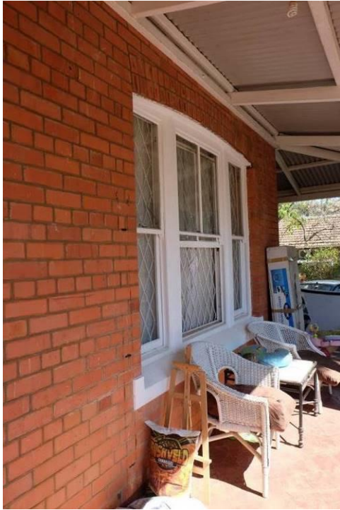
Fig. 13 & 14_Original wooden sash windows towards the verandah (left); original wooden main entrance door (right) (Source: tsica heritage consultants, 22.09.2020)
