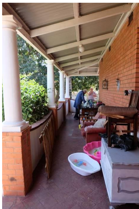
Fig. 18 & 19_Verandah wrapped around the corner (left); Verandah roof is supported by a row of columns (right) (Source: tsica heritage consultants, 22.09.2020)
