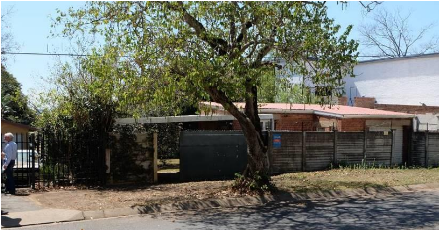
Fig. 50_Single storey red brick outbuilding which was used as storage and garage along Carbis Road (Source: tsica heritage consultants, 22.09.2020)
