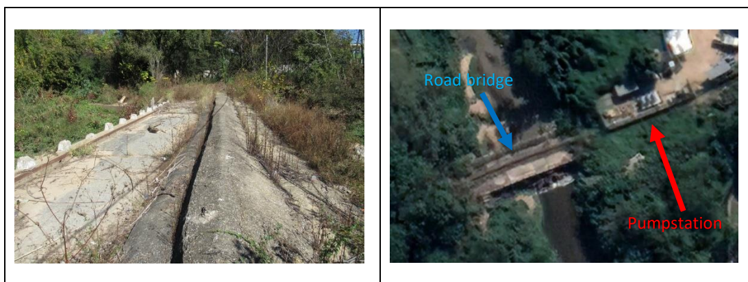
Figure 13. View of the old concrete road bridge
