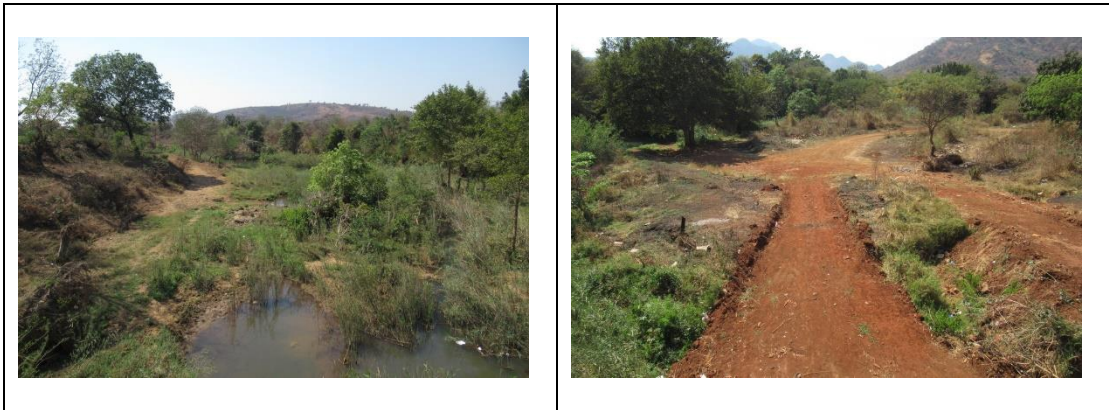
Figure 9. Bridges and riverbanks
