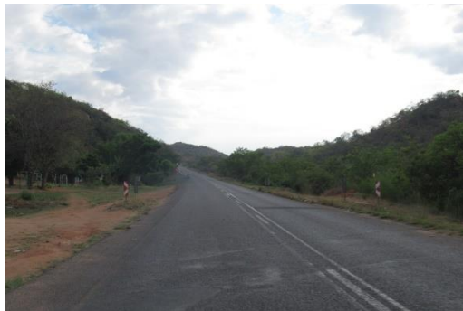
Approach to the cutting
