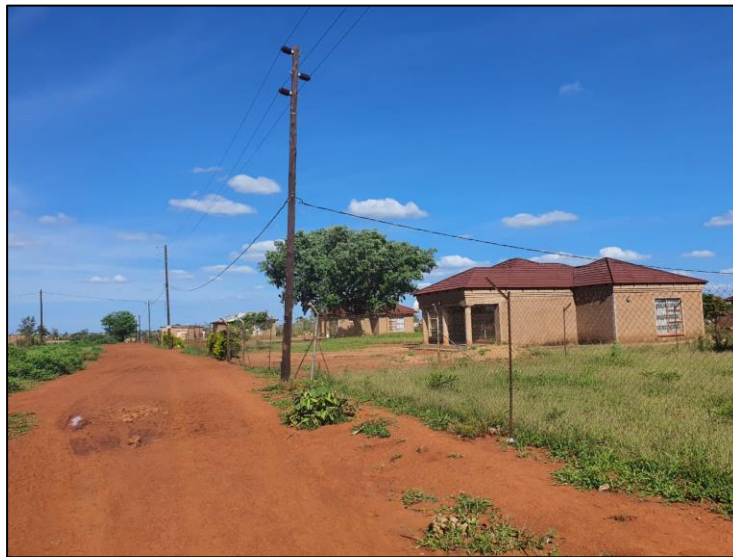
Figure 3-13: View of the alignment of Deviation 3 through Maphophe.
