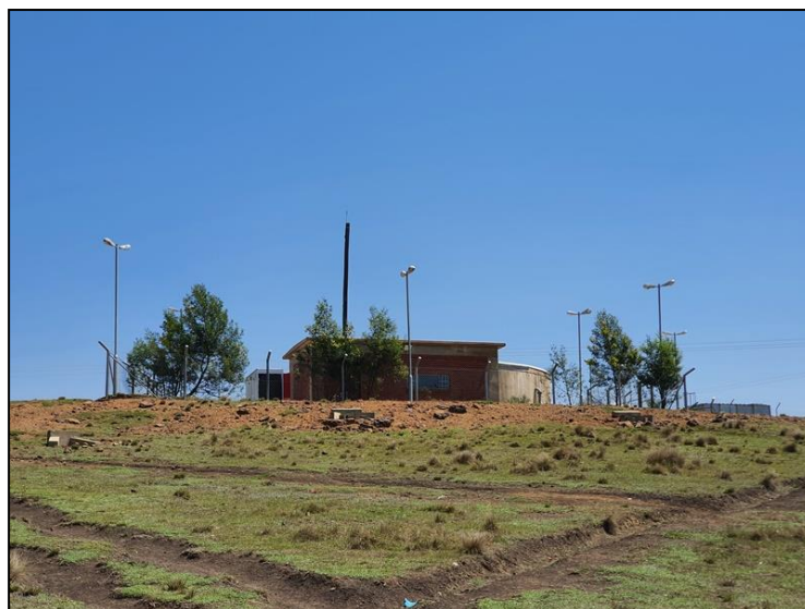
Figure 3-2: View of the BPS2 reservoir at the northern offset of the alignment.
