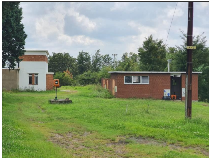
Figure 3-2: View of the Standerton WWTW along the proposed alignment for the preferred pipeline route.
