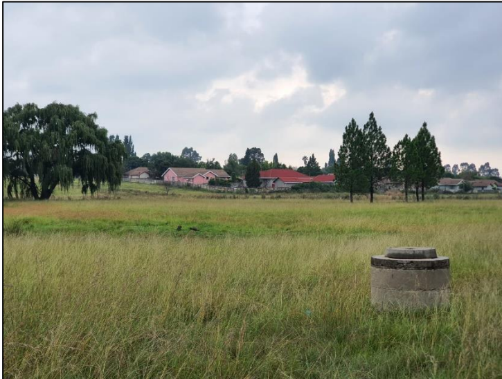
Figure 3-7: View of a drainage line along the alternative 1 alignment for the pipeline route.
