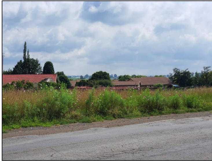
Figure 3-9: View of the proposed alignment for the preferred pipeline route along the R39 road in Standerton.
