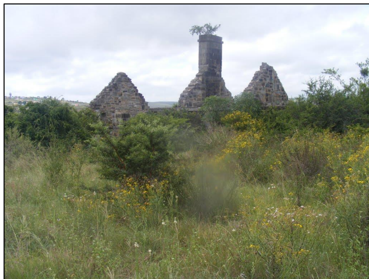
Figure 4-6: View of the remains of Fort Murray along the Buffalo River ( http://www.artefacts.co.za/main/Buildings/bldgframes.php?bldgid=10397 )
