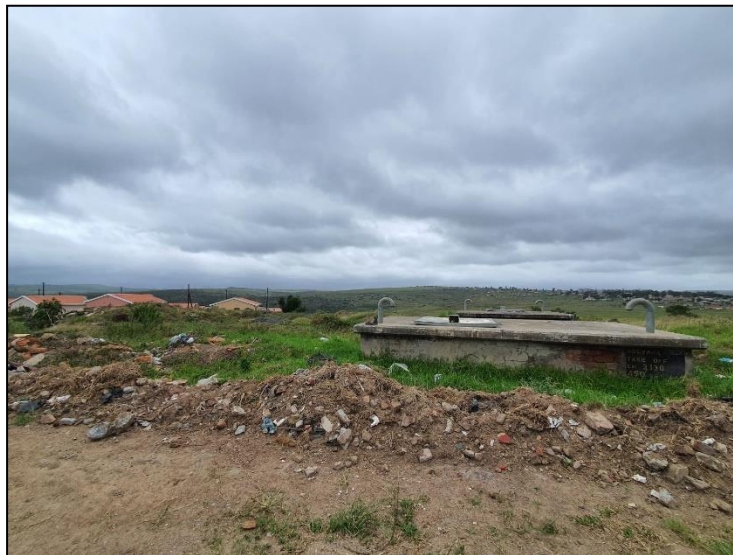
Figure 3-1: View of the south western offset of the proposed pipeline alignment in Phakamisa.
