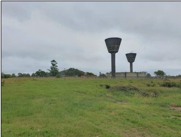
Figure 3-6: View of the north eastern offset of the proposed pipeline alignment in Berkin.
