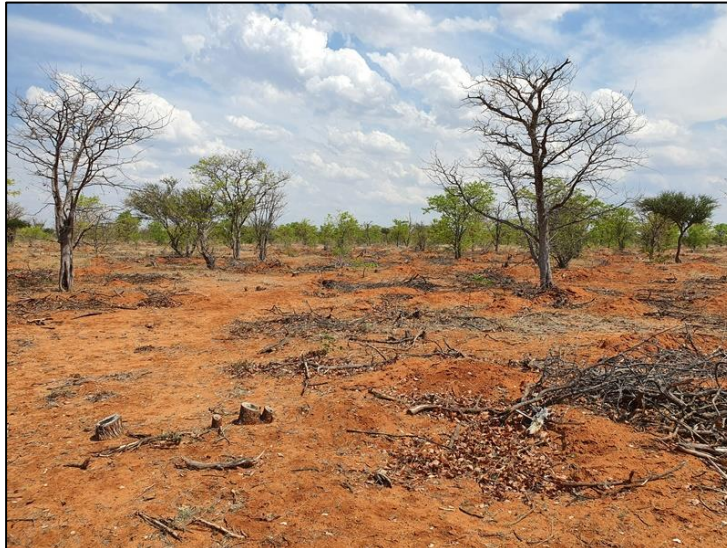
Figure 3-6: View of ripped and excavated Mopaneveld in a western portion of the project area.
