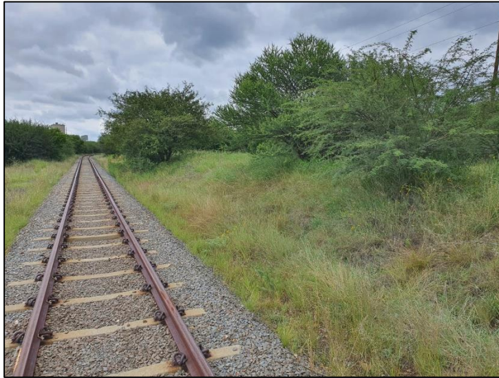
Figure 4-6: A Transnet railway line forms the southern boundary of the project area.
