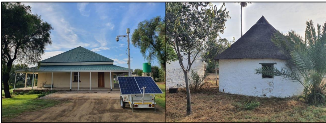
Figure 5-20: View a historical farmhouse and rondavel at Site Exigo-VSP-HP04.
