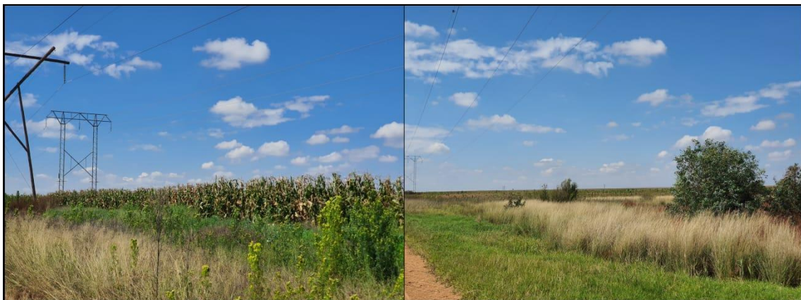
Figure 3-3: View of sections of the project corridor through cultivated lands.
