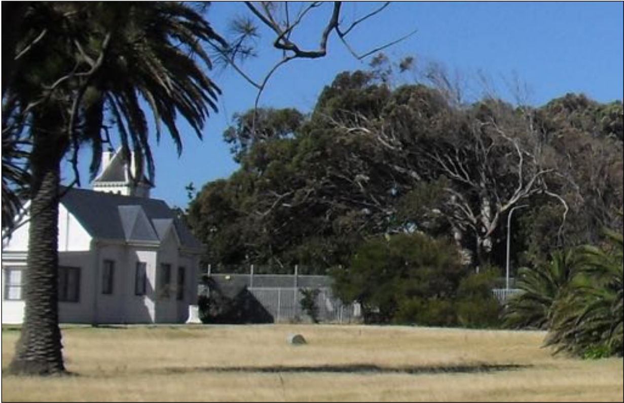
Figure 20: The southern façade of the pre-1891 Victorian house occupying the north-eastern corner of study area in 2009. (Jim Hislop, 2009)
