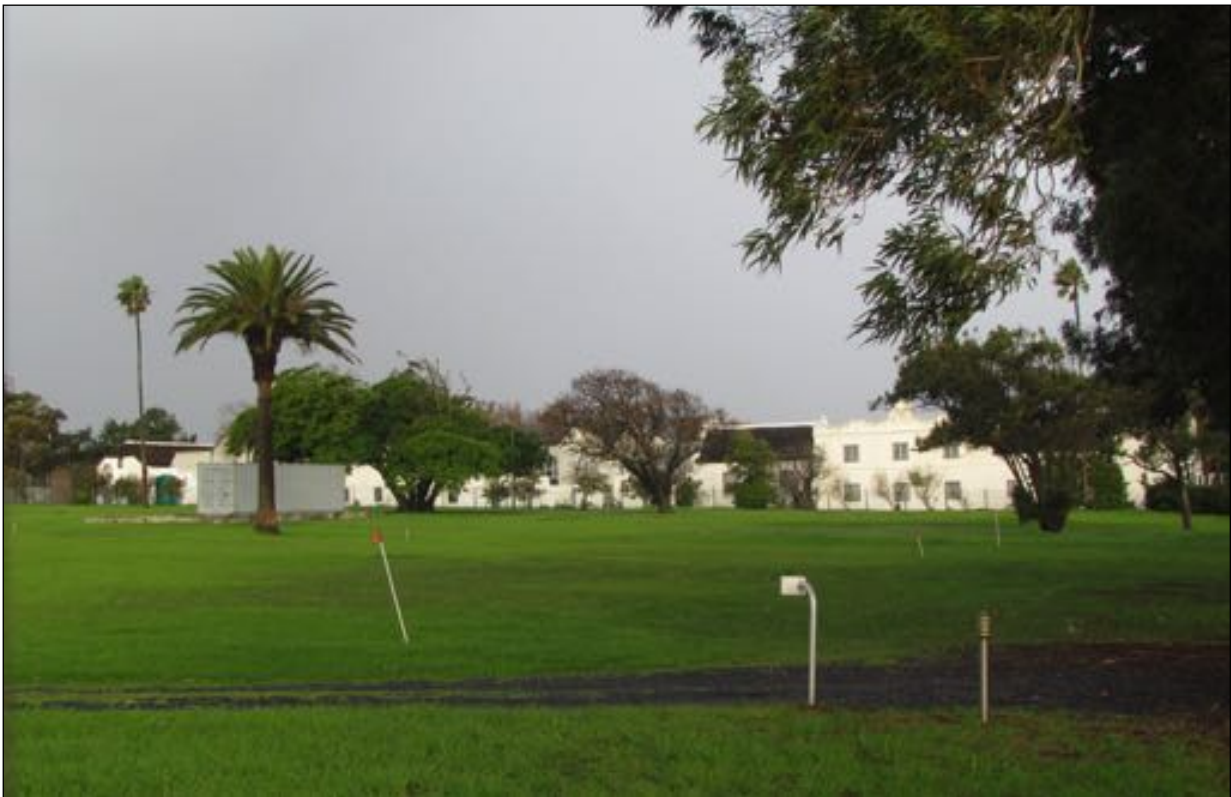
Figure 43: Looking south across the central part of the study area towards the 160-metre-long Valkenburg opstal, with the platform and container at left. This unobstructed view of the opstal is still recognisable when compared to the 1834 Bowler artwork (Figure 5). The restored rear barn can be seen at centre left, and the restored wavy parapet section of the manor house is at right.
