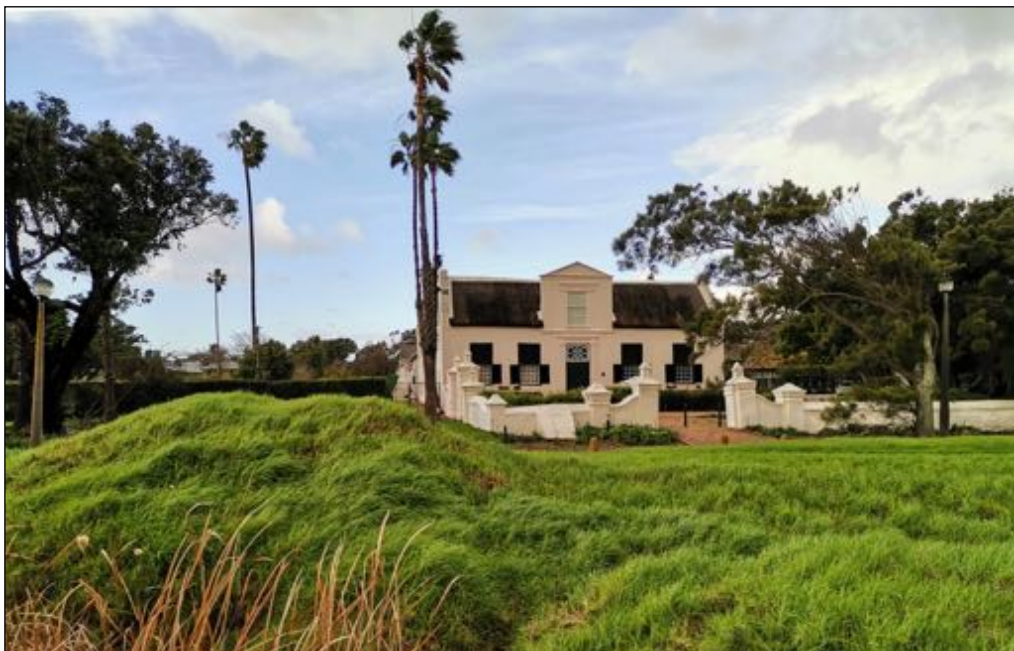
Figure 14: The 'front' façade of the Grade II-listed Valkenburg opstal, facing west towards Table Mountain and the Liesbeek River. Restored in 1984, it is now occupied by the Protea Hotel Mowbray. The boundary hedge of the study area is seen at centre left. (Jim Hislop, July 2021)
