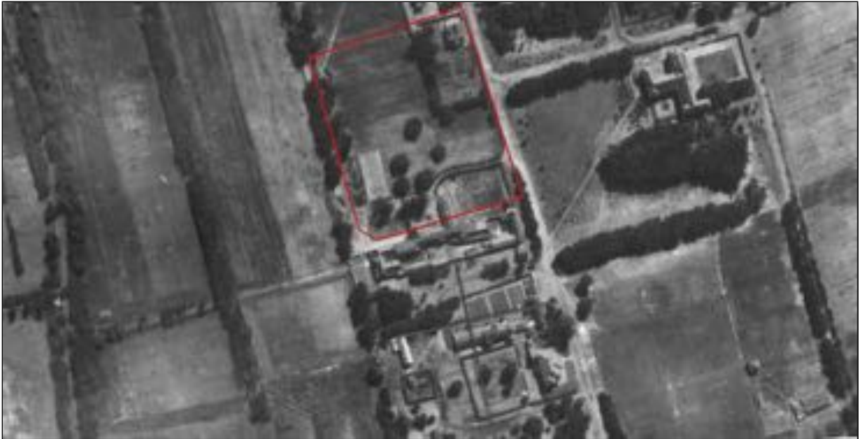
Figure 28: By 1934, according to the aerial photographic survey of that year, the Valkenburg opstal complex and werf (then still relatively intact) had by this time been extended with a north-facing wing extending into the subject area, with a curved access pathway leading to this wing from the east. In the north-eastern corner of the study area, the Victorian house can be seen, with an enclosed formal garden extending southwards. Various mature trees can be seen on the property, as well as a rectangular raised area in the south-west corner. A line of trees marks the perimeter of the subject area to the west along Liesbeek Road. (Chief Directorate: National Geo-spatial Information: 282_001_19394)
