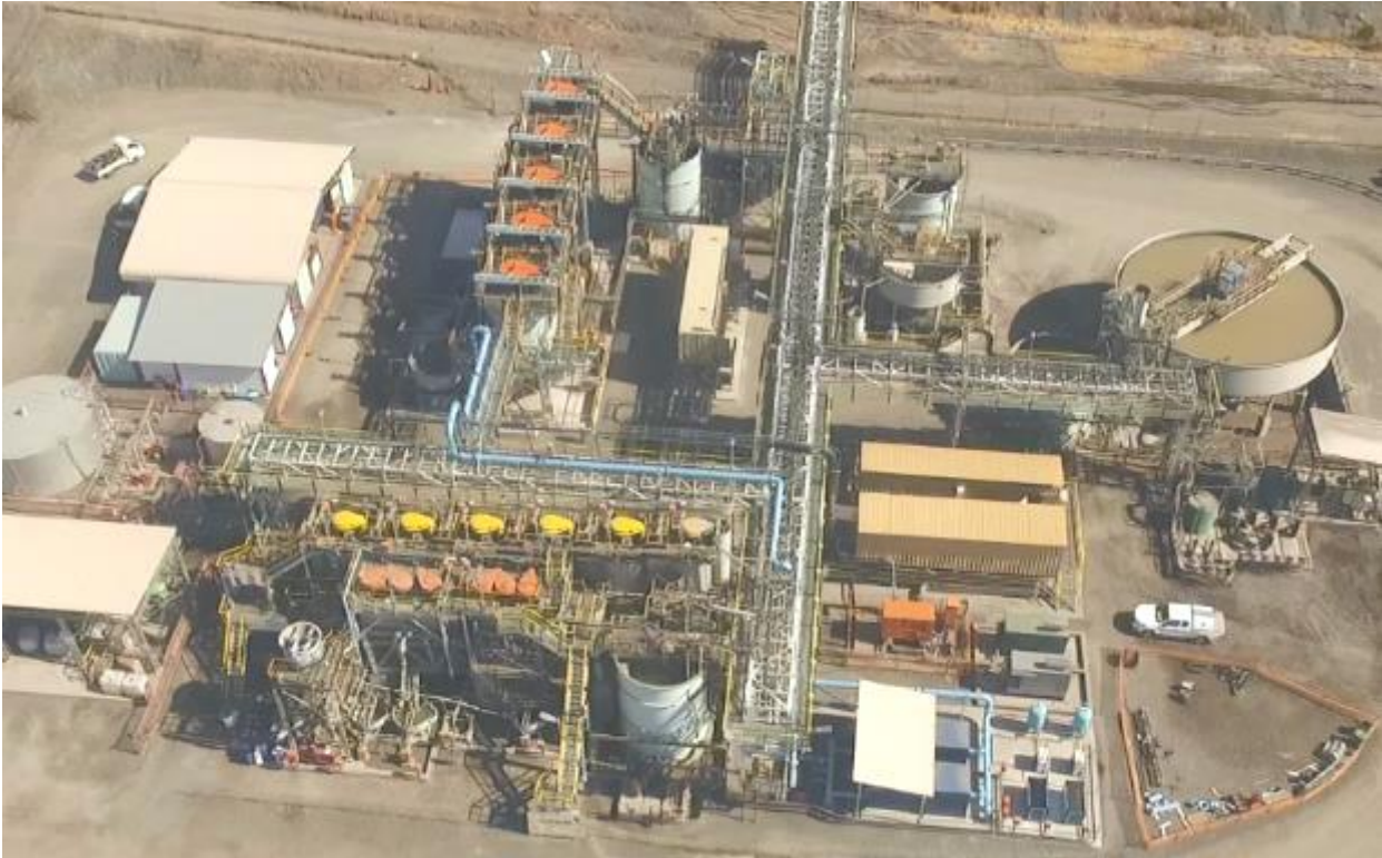
Figure 5-1: The existing PGM plant
