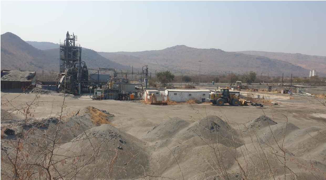
Figure 5-2: Site proposed for the FCR plant showing existing stockpiles and the chrome recovery plant
