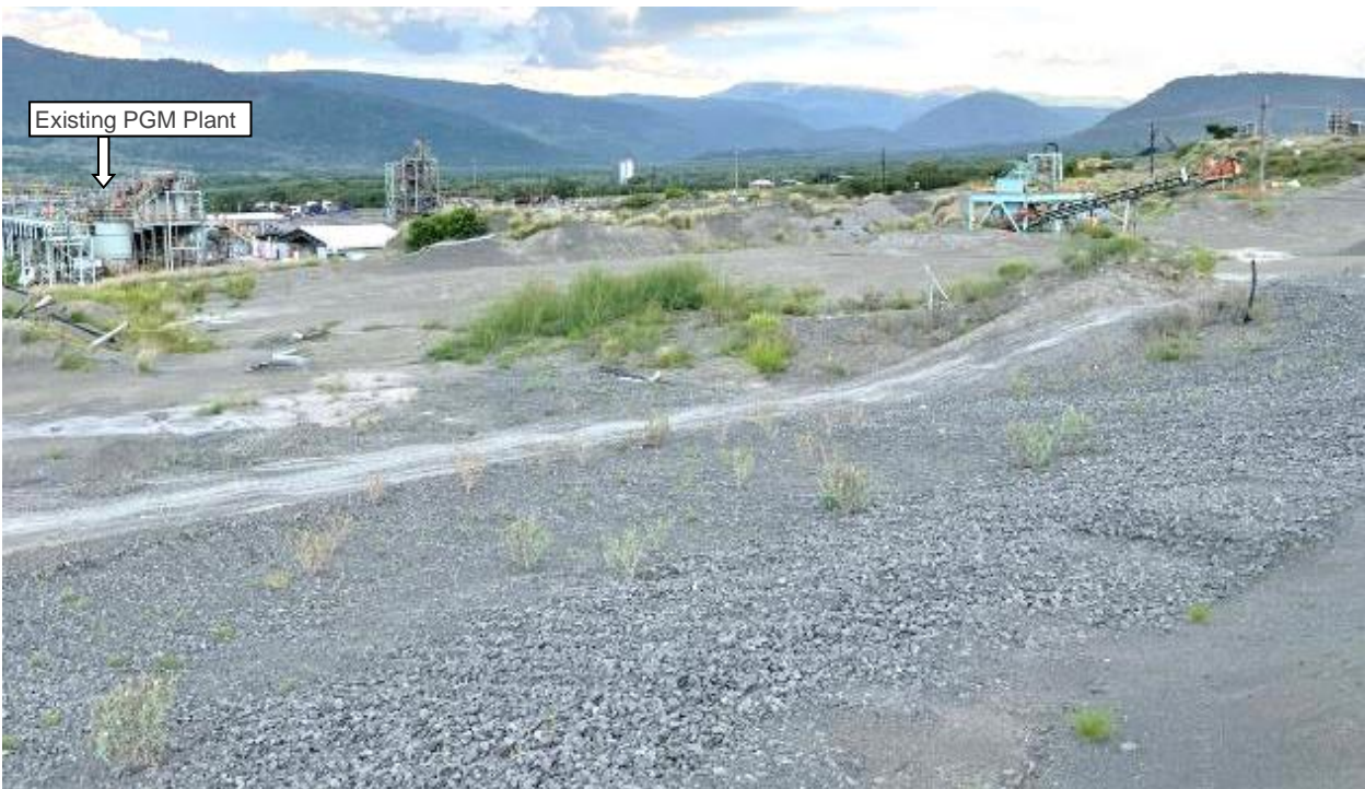
Figure 5-6: Site proposed for the PGM plant – view towards the east
