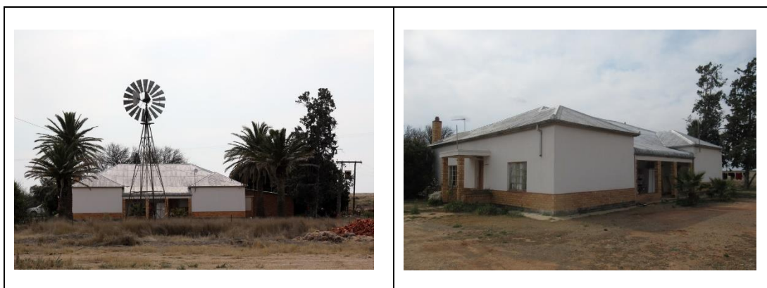
Figure 19. Views of the main house at the farmstead
