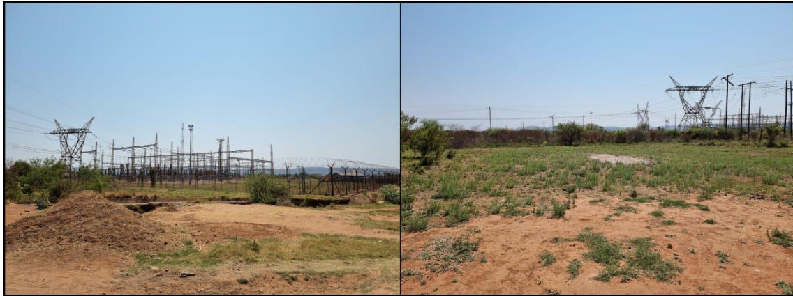
Figure 3-1: View of general surroundings in the project area with the ESKOM Warmbaths Transmission Substation (left) and the exiting ESKOM Powerline servitude (right) visible.
