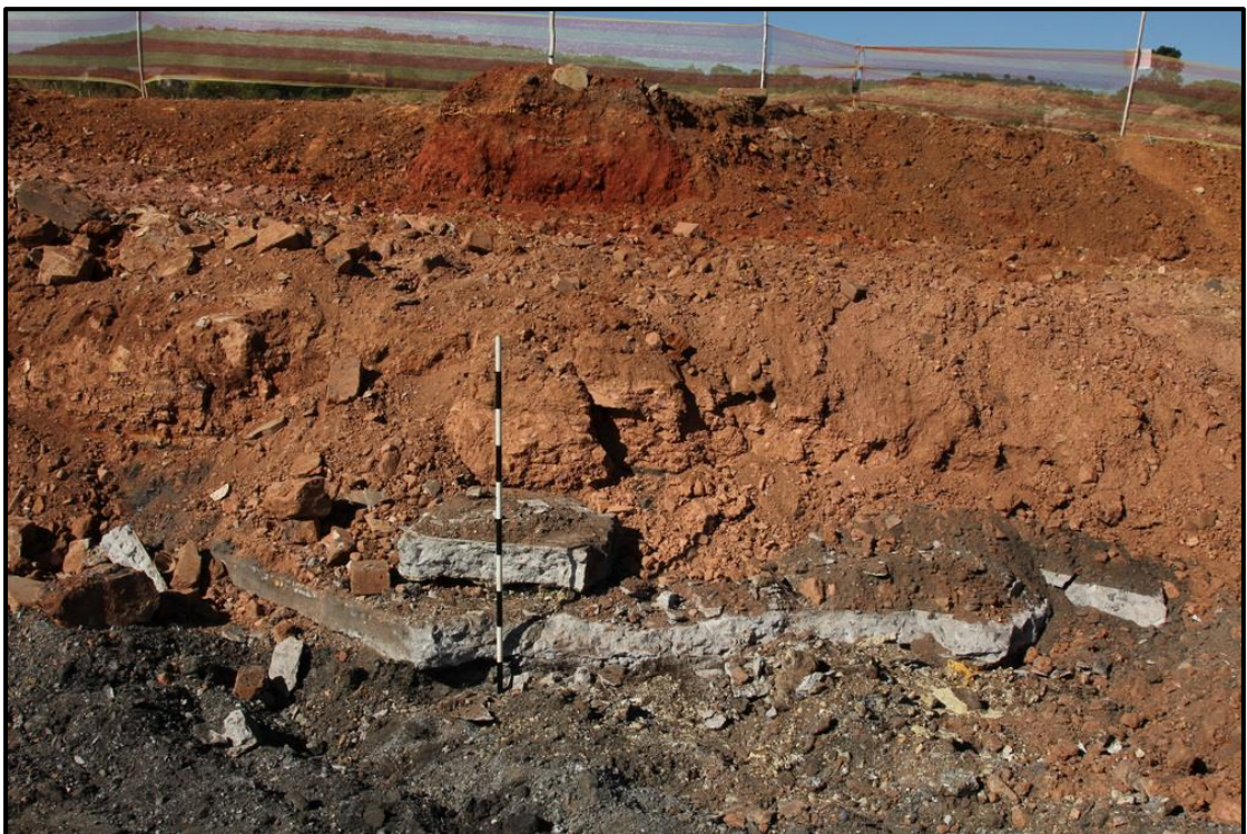
Figure 16. Showing the depth of the rubble back-fill
