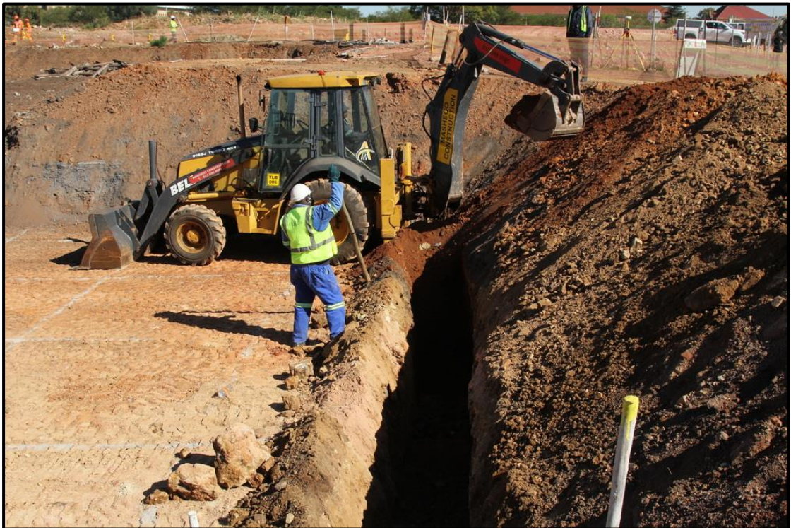
Figure 15 Image indicating the depth of the building excavations
