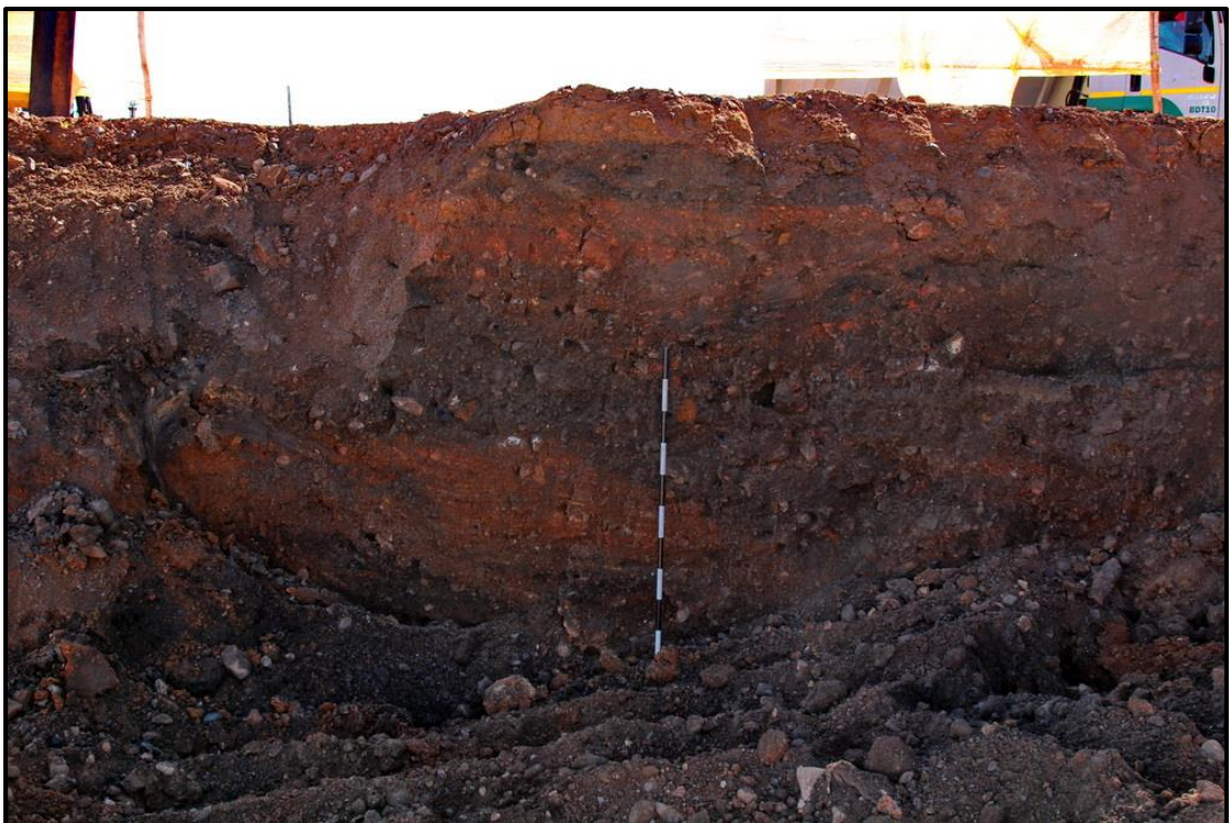
Figure 18. Showing the depth of the back-fill
