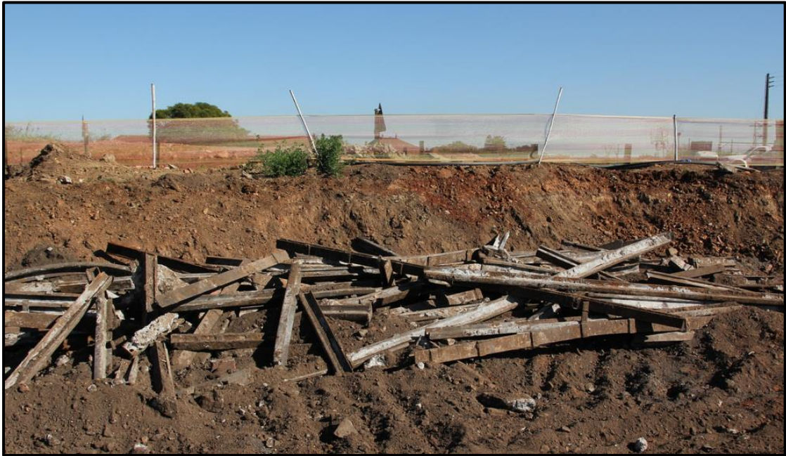
Figure 19. Showing the depth of the back-fill with rubble
