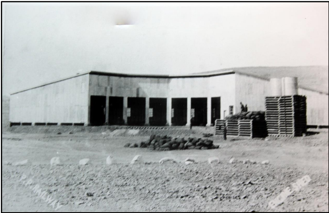
Figure 5. The Pretoria-Pietersburg round house under construction, pre-1899
