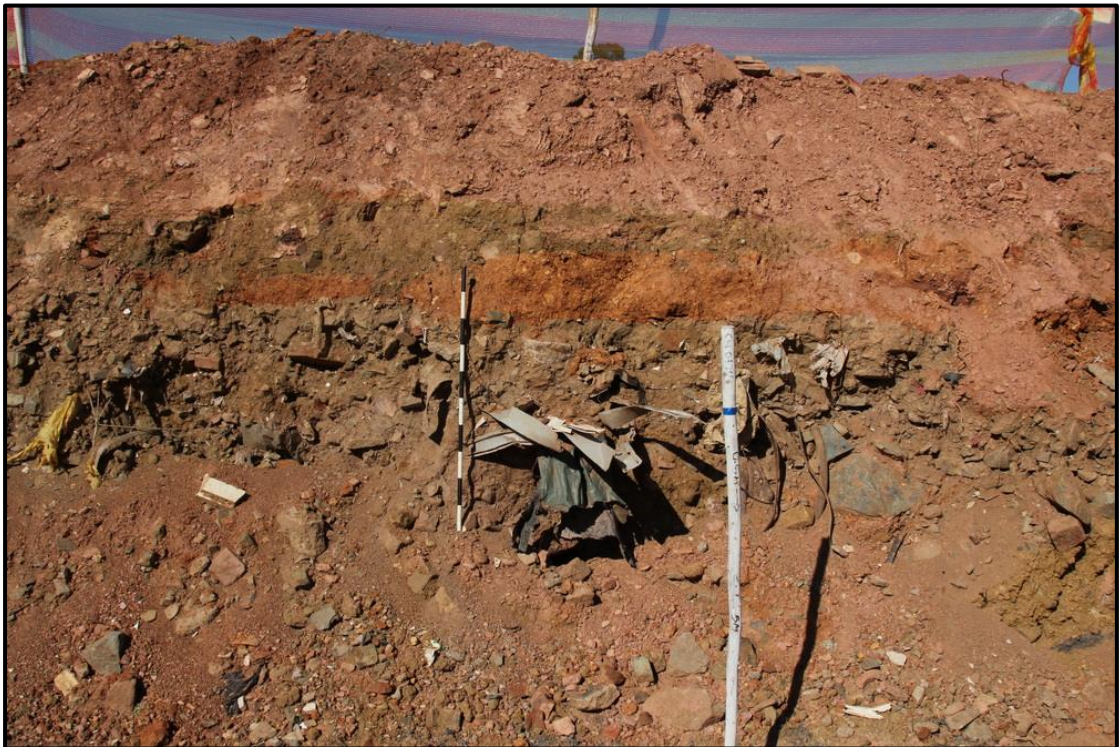
Figure 17. Showing the depth of the back-fill
