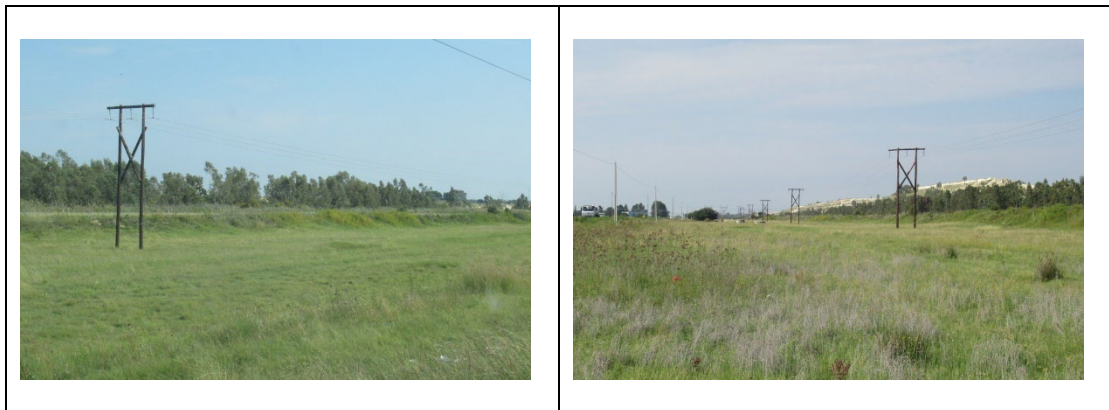
Figure 6. Views along the power line route
