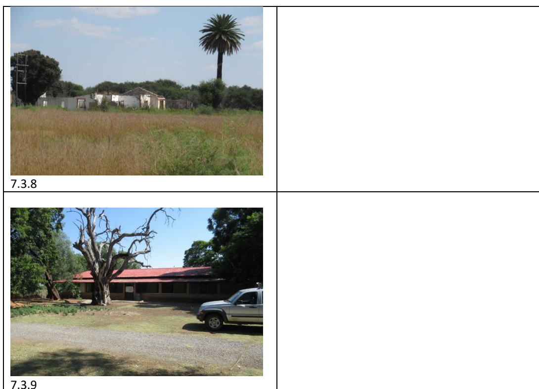
Figure 15. Views over the old structures
