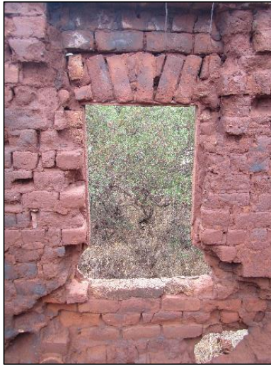
Figure 41: View of Window frame.
