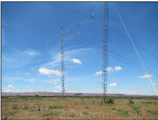
Figure 3: View of the existing power line and servitude near the R31, south of Kuruman.
