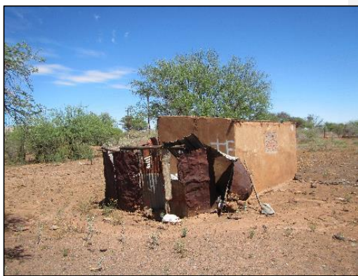
Figure 29: General view of structures at K025
