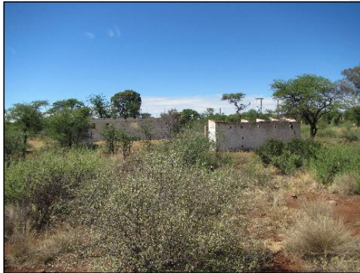
Figure 27: View of abandoned buildings
