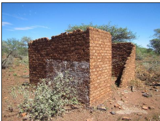
Figure 28: General view of the identified structures at K025
