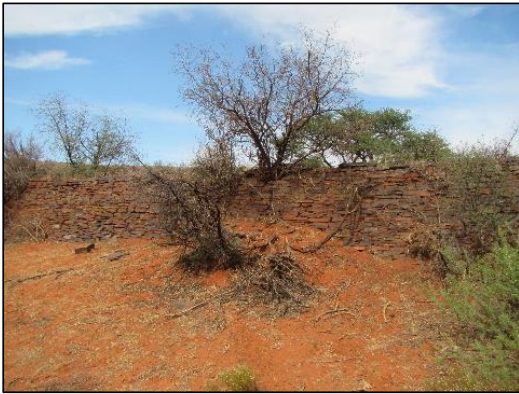
Figure 34: Remains of anti-erosion walls.
