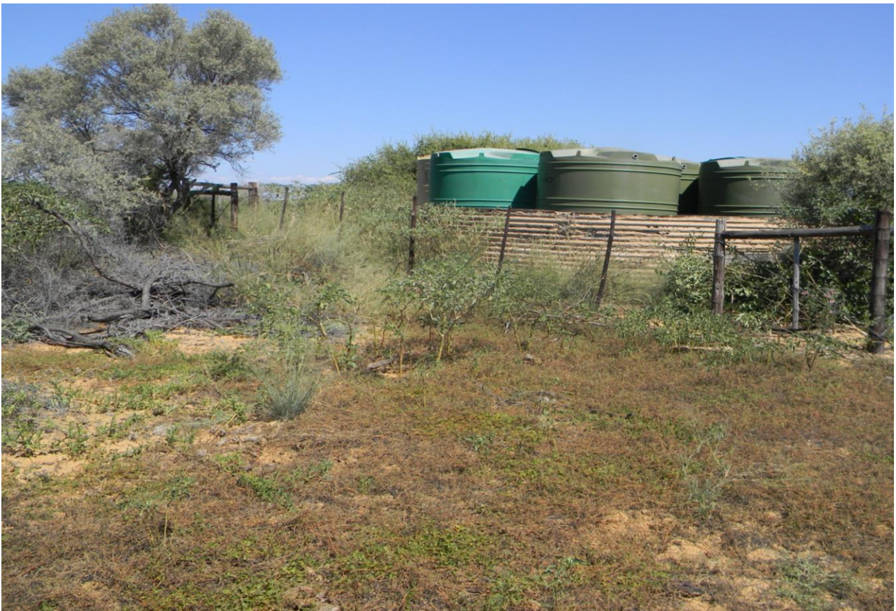
Plate 6: Photo 6: View of water tanks within the proposed prospecting site (Photograph © by Author 2020).
