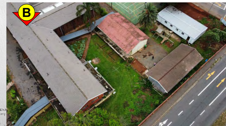
The additional classrooms are of temp materials, timber & asbestos, a prefab panel and tiled structure, and a container structure that have been used. The asbestos structure has been demolished.
