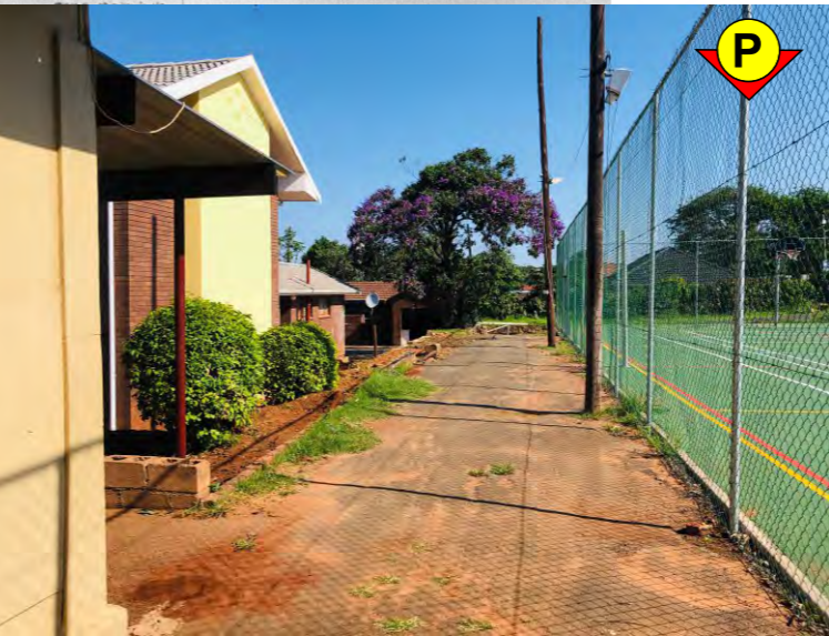
ORIGINAL STRUCTURES- These were constructed out of a face-brick exterior with steel casement windows. The arch detailing with the shallow triangular arch is reminiscent of Anglo-Saxon styling, with the accent detailing on entries and canopies now painted yellow, similar to the timber structure of the added classroom block. The outbuilding is still in reasonable condition, but did not have any striking character or architectural depth, but also needs some maintenance work on it. The addition of the combination court is recent, and is covers the west roadside elevation of chapel building
