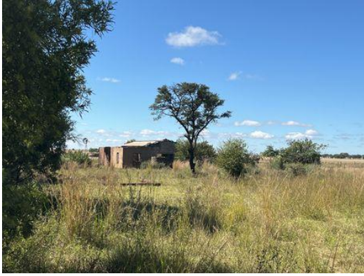
Figure 21 - View of some of the structures at D1-001
