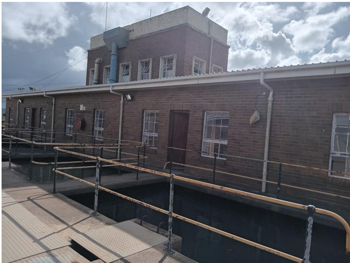
Figure 27: View of two buildings to the north of the Main building at the water treatment area
