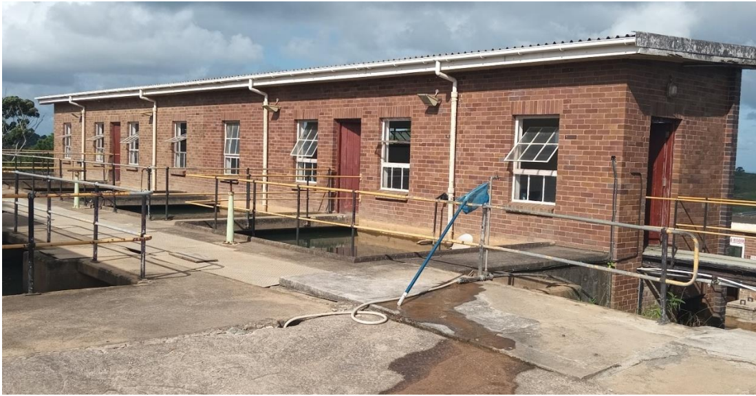
Figure 26: View of Building southeast of the Main building, from the Water treatment area
