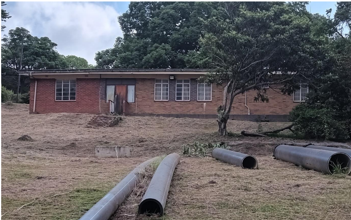
Figure 33: View of another building located to the north of the waterworks buildings
