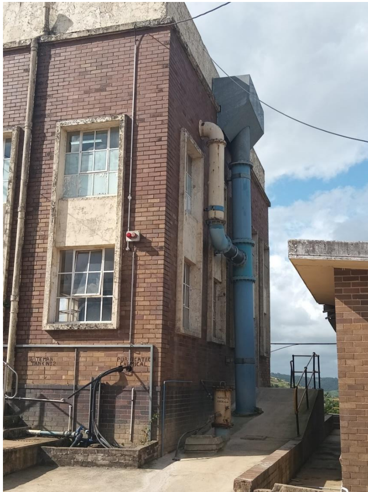
Figure 28: View of the second building located north of the Main Building
