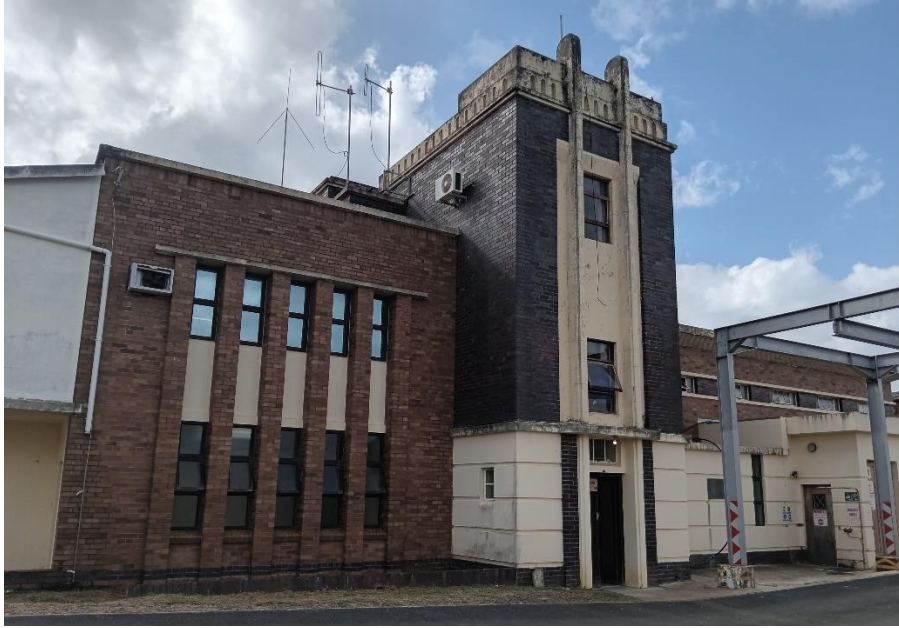
Figure 22: View of the main building showing the strong vertical elements reminiscent of the Art Deco style, although the yellow and purple brickwork indicates a more likely date of c1940s-1950
