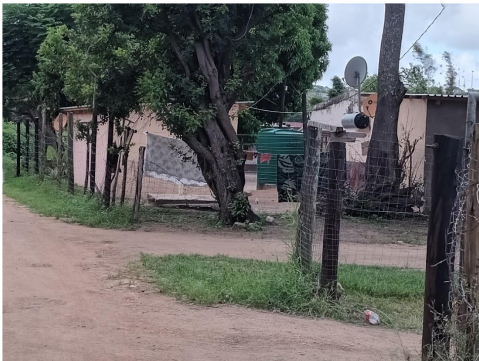
Figure 9: View showing some of the existing houses along the southern section of the pipeline corridor
