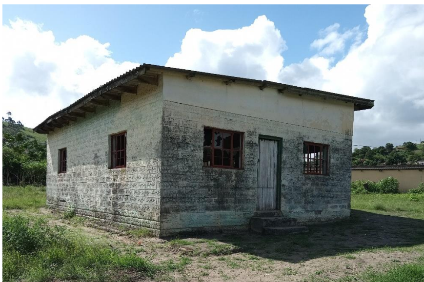
Figure 18: View of the old house at UMZ-P02
