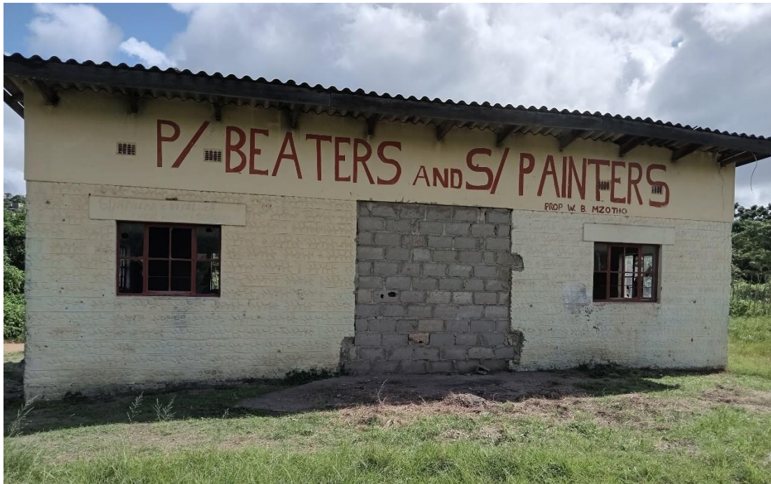
Figure 19: View of the panelbeaters shop, showing that the entrance has been blocked with concrete bricks
