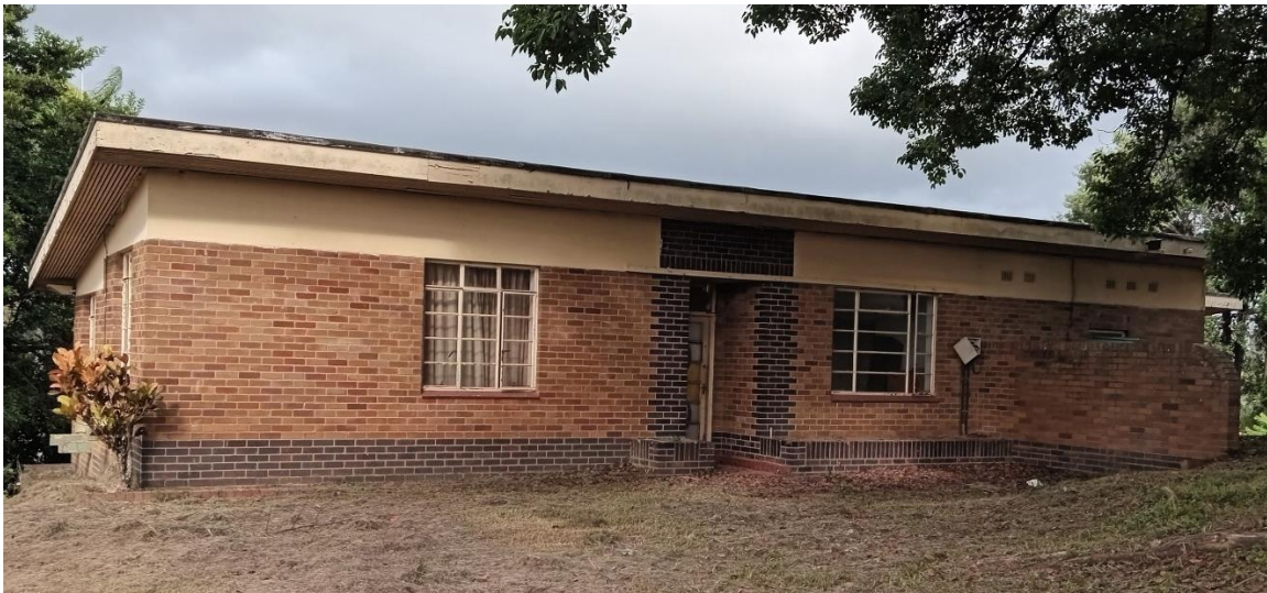
Figure 31: View of house situated near to the entrance to the Water Treatment Plant, showing the similar brickwork to the main complex
