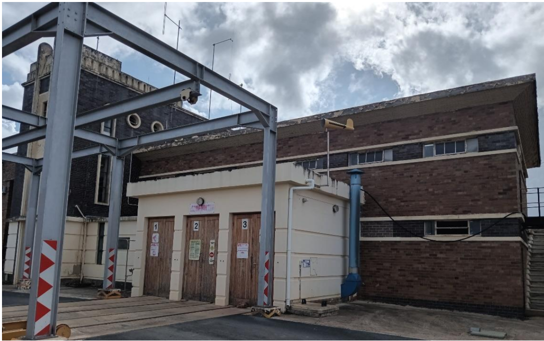
Figure 24: View of East wing of main building
