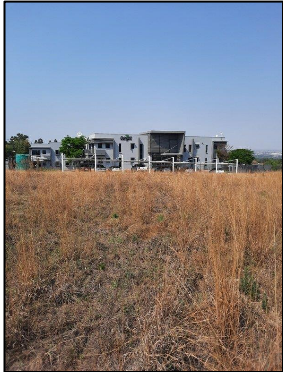
Figure 7.8. Small office complex situated west of the project area.
