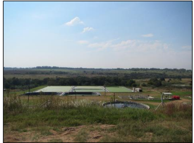
Figure 7: View of the water treatment facility
